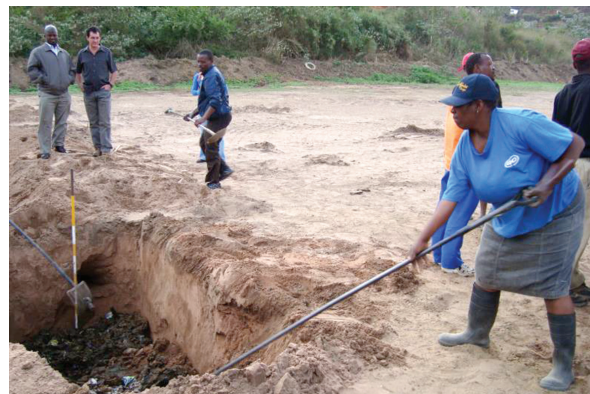
Sludge burial in progress.
