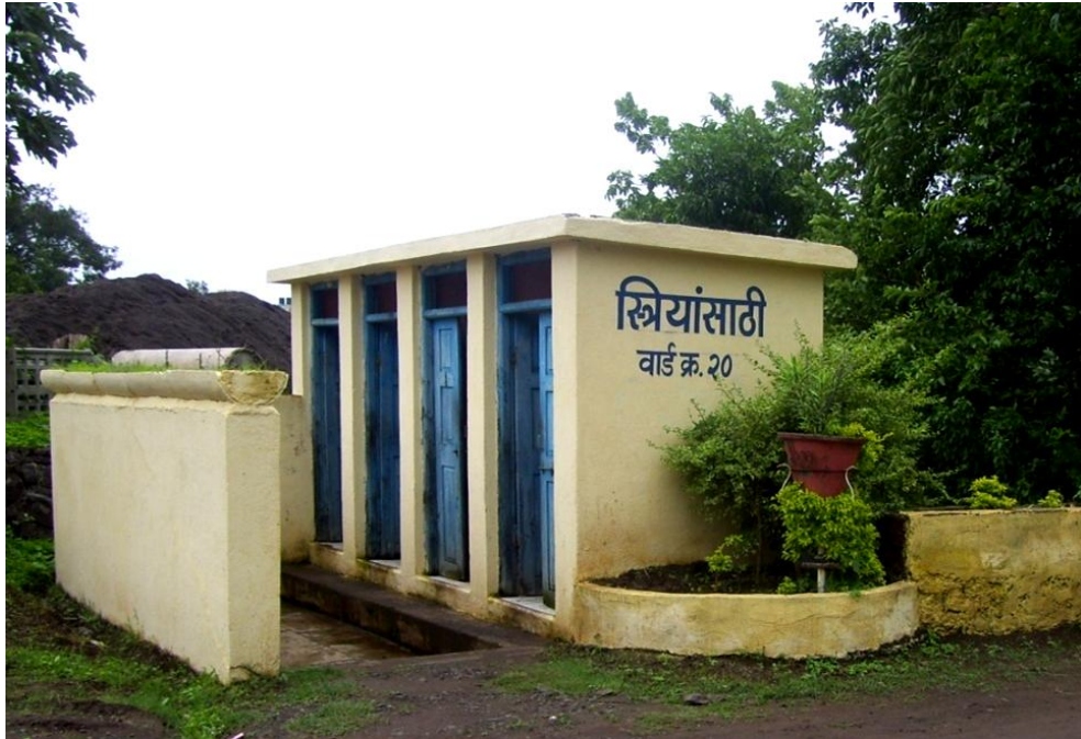
The toilets are well maintained and accessible in non-slum areas too.
