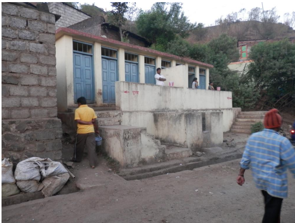
One of the community toilets built by the SMC.
