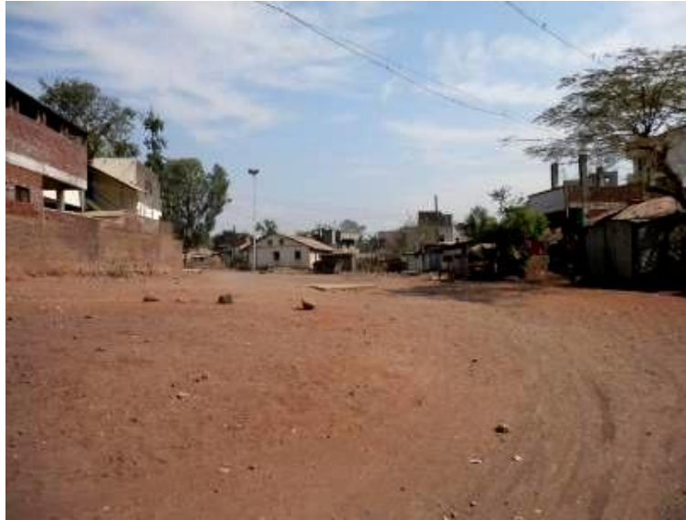
An open defecation space cleared of debris and garbage.
