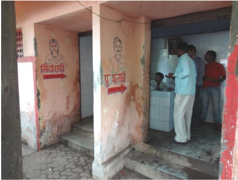
A public toilet with separate entry for male and female users. The city has similar arrangement for all its community toilets.
