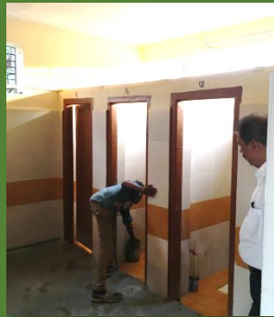
Community toilet at Chopda. Clean surroundings, ample of light, air and space inside the toilets, Provision of room for caretaker
