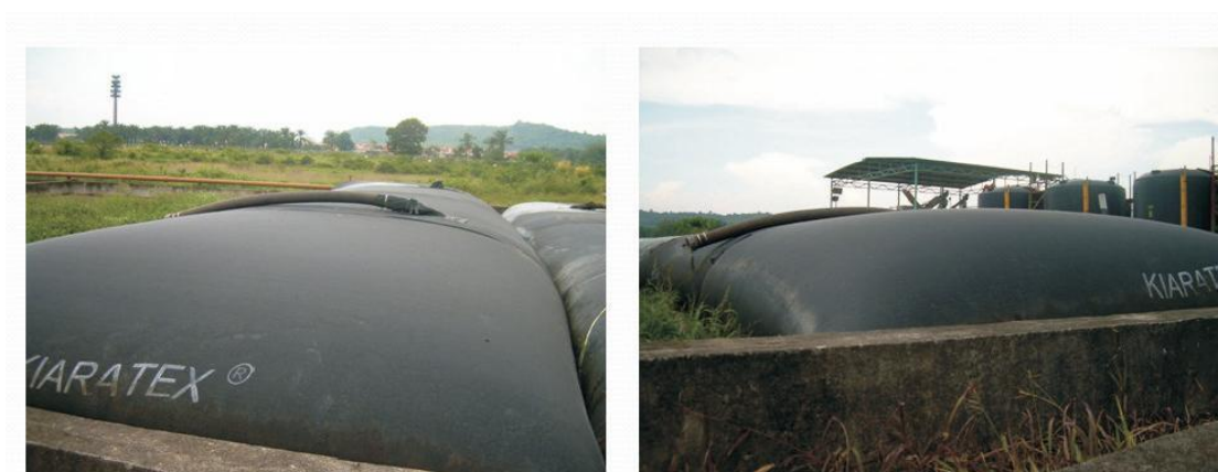
Figure 3.8.5: Geo-tube when it is filled
