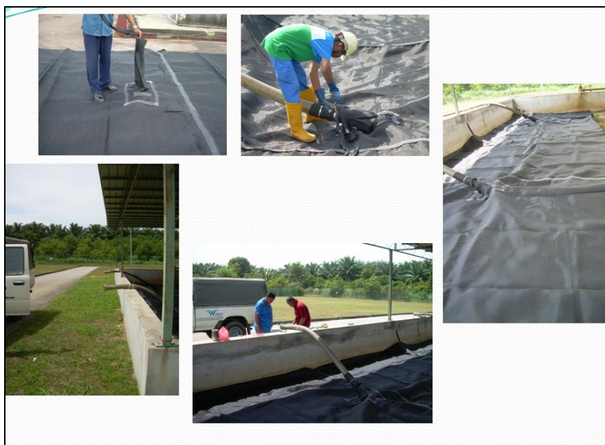
Figure 3.8.4: Pumping of Sludge into the Geo-tube/ Geo-bag
