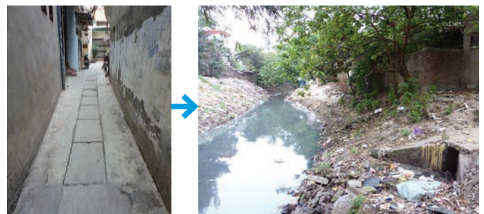
Figure 2.3: Combined drainage systems in Hanoi, discharging to open channel
