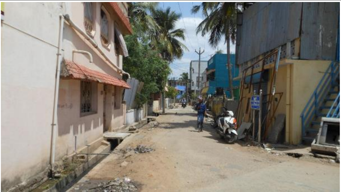
Plate 3-12: Surface Storm Water Drains in Pammal
