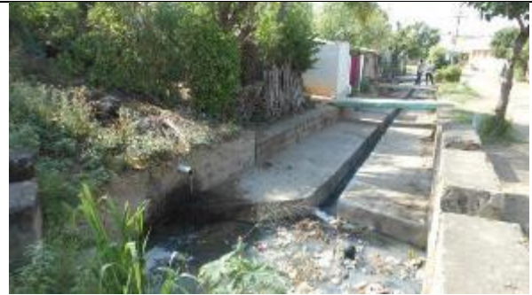
Main Storm Drain of Narasimhanaicken-palayam
