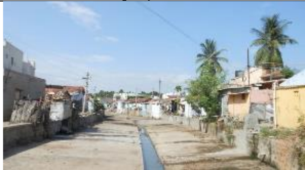
Main Storm Drain of Periyanaicken-palayam
