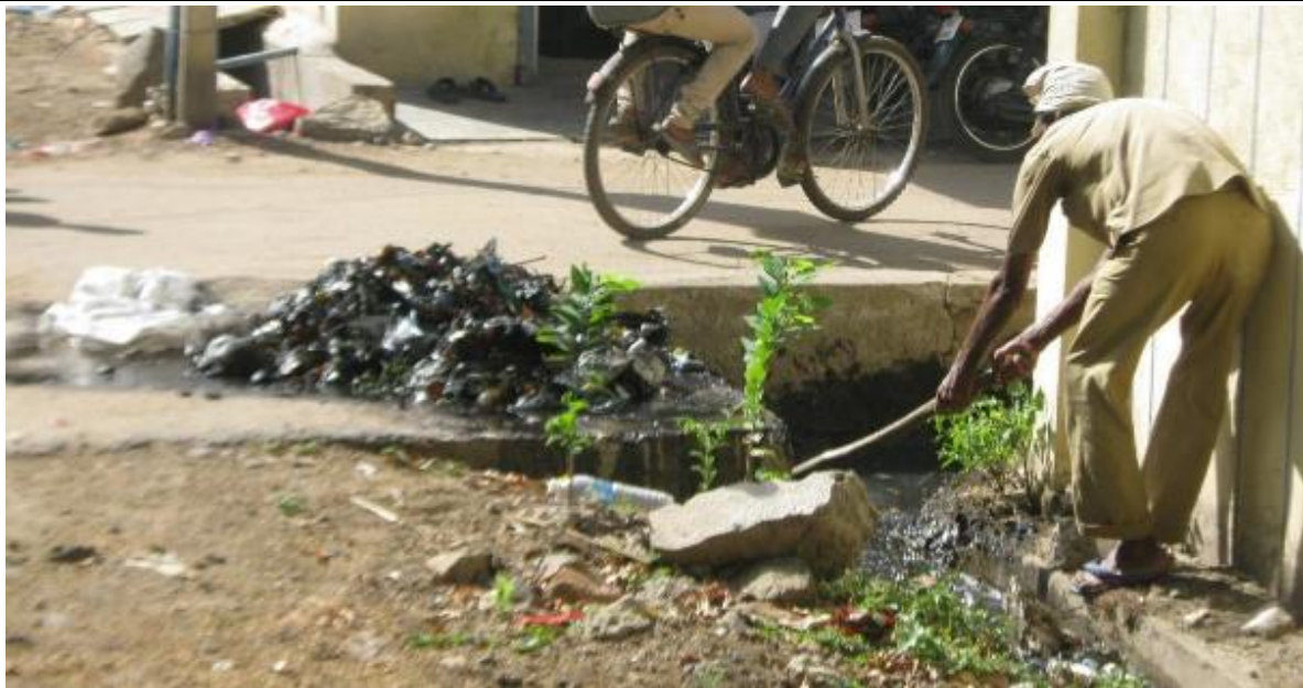
Plate 3-9: Drain cleaning by sanitary worker in Pammal
