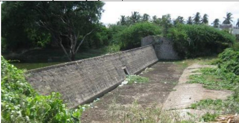
Check Dam on the Kousika River in Narasimhanaicken-palayam
