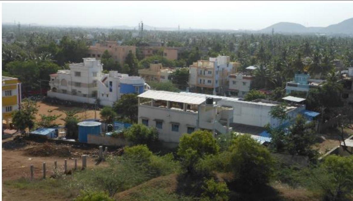
Plate 3-8: Biomethanation plant for treatment of food waste in Pammal
