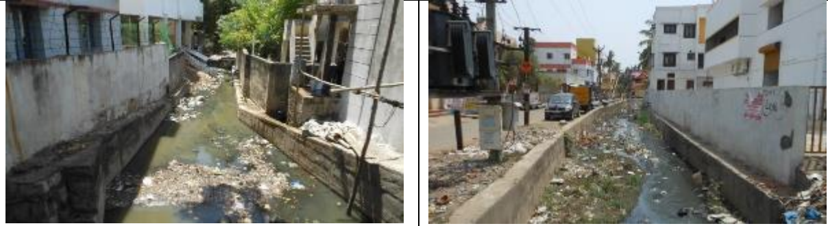
Main storm water drain from Thirupunanthal
