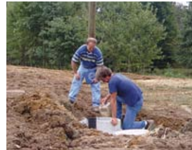
Inspecting a septic system. Photo: Kentucky Department of Health
