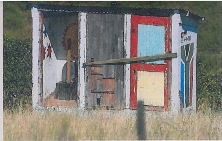
IN DIRE STRAITS: Bulugha Farm School, situated just outside East London, is one such school that had to make do without proper toilet facilities. The school, which has 250 pupils enrolled, made use of a single pit latrine while other pupils were forced to relieve themselves in the bushes PICTURE: MARK ANDREWS
