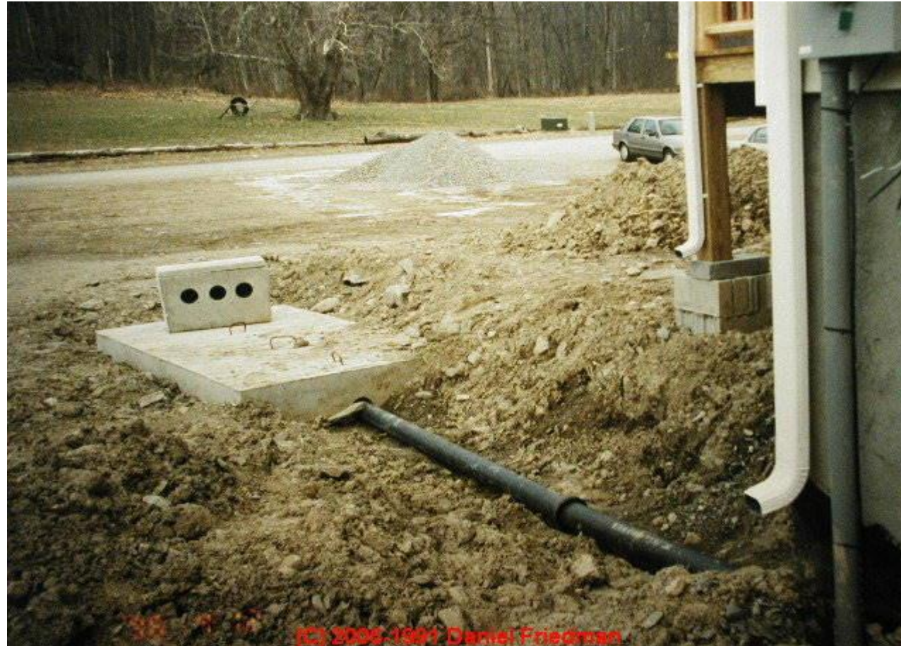
Piping and connecting to toilet pan
