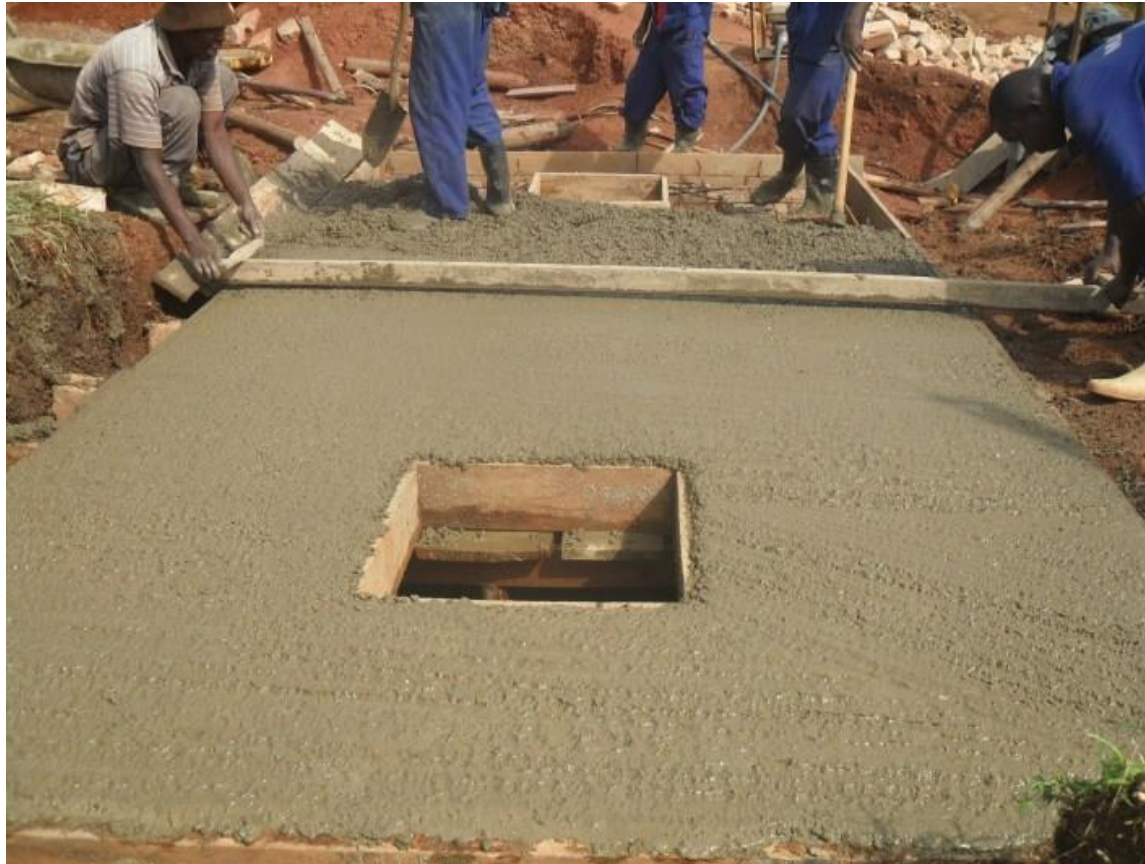
Top RCC with Opening for Manhole
