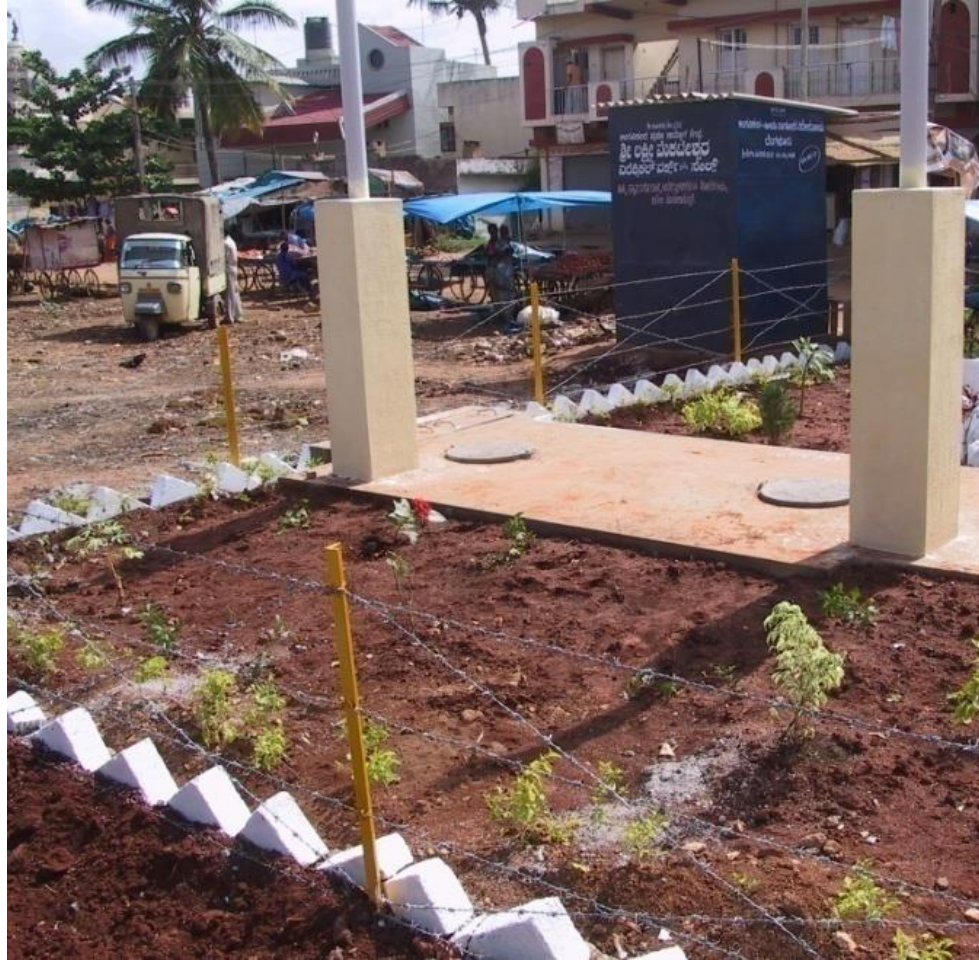
Backfilling & Clearing of Debris
