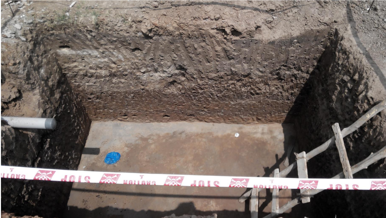
Leveling of the base
