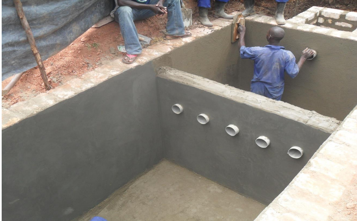
Waterproof plastering of walls
