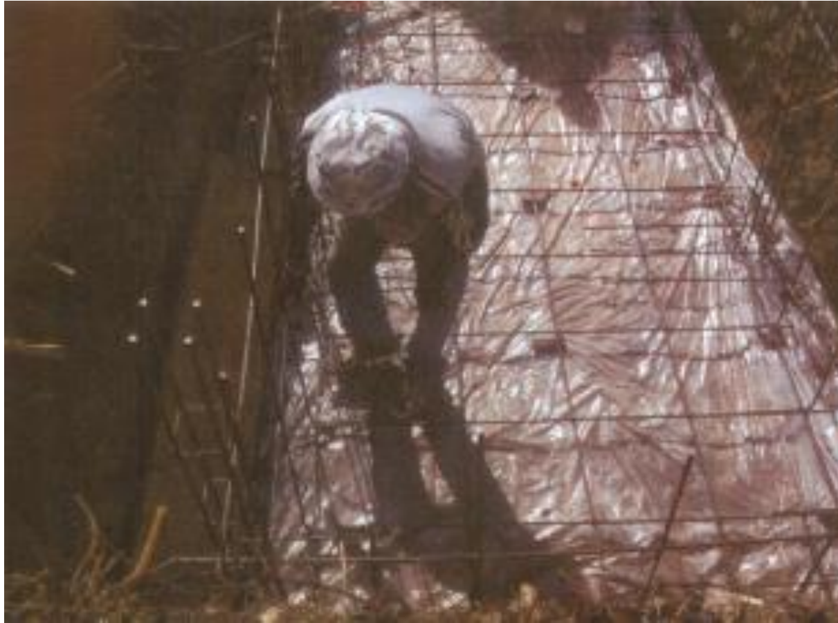
Leveling of the base
