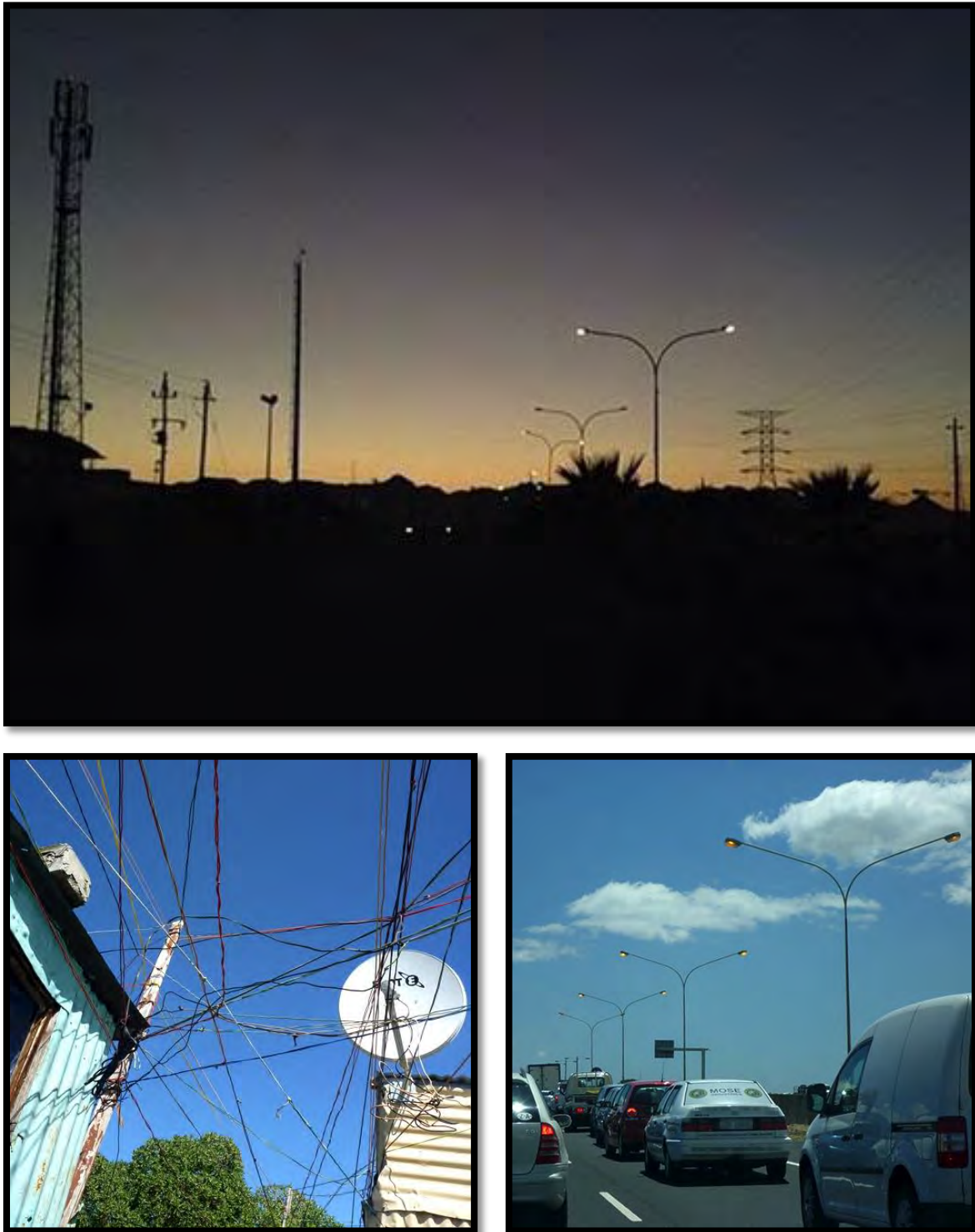
Figure 37: Area lighting in BM Section at 6:00 (top, Norvixoxo, 6 April 2014). A tangle of overhead wires from illegal connections in BM is featured on the bottom-left. The majority of residents living at the back of BM arranged ‘informal’ connections with households near Lansdowne Road that had pre-paid boxes. The ‘suppliers’ said that their ‘customers’ paid an average of R125 per connection. On the bottom-right are mast lights left on at 14:20 on the N2 near Khayelitsha (Taing, 2 May & 4 February 2013).
