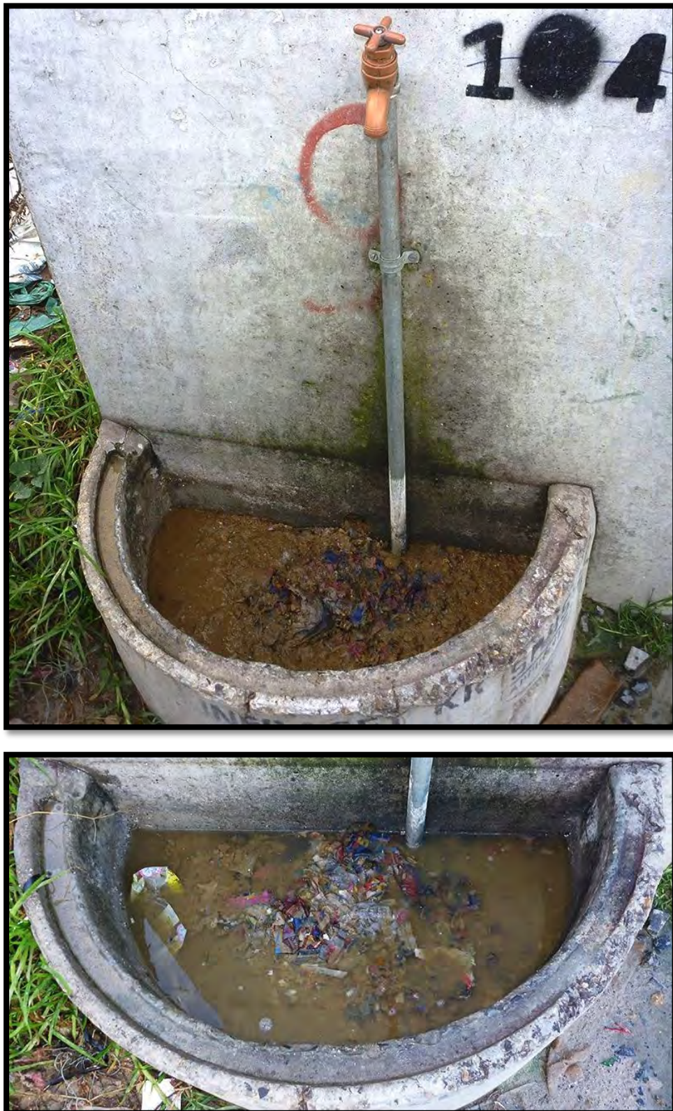
Figure 40: Limited drainage has supposedly resulted in the contents of night pails being dumped into the drains of taps that provide clean water in BM Section (top). I noted that the waste remained there for several days, despite there being janitors to clean shared water and sanitation facilities in BM (bottom) (Taing, 14 & 16 February 2013).
