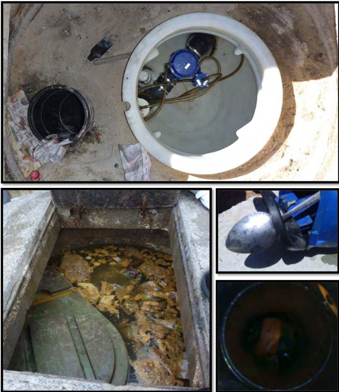
Figure 21: Clockwise from the top: (a) A collection chamber in Kosovo’s vacuum system, with the sump on the left and the sensor unit on the right (Taing, 15 April 2011); (b) a damaged interface valve diaphragm (Cornelius, 26 June 2009); (c) a brick in the sump (Cornelius, 28 February 2010); and (d) a flooded chamber (Taing, 7 June 2010).
