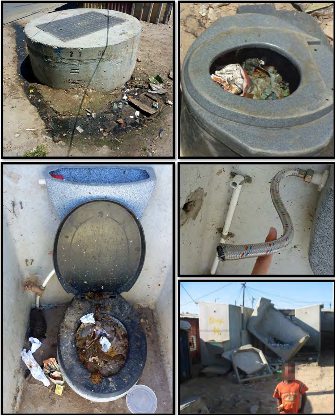
Figure 22: Clockwise from top: (a) sewage seeping from a collection chamber (Taing, 29 November 2010). While (b) container toilets are unsightly and smell, Kosovo residents preferred them to the ineffective vacuum toilets because the contents of the plastic containers did not seep into the surrounding environment. Residents, who were dissatisfied with the malfunctioning system, also (c) cut water supplies of units to deter usage (Taing, 11 November 2010) and (d) destroyed toilets in protest (Pan, 30 May 2010). But, as (e) the photo of a full but disconnected toilet indicates, some nevertheless continued to use the vacuum toilets (Taing, 15 April 2011).
