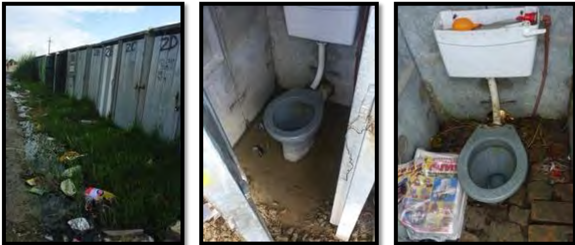
Figure 44: Toilets tended to be located in open spaces that oftentimes were undesirable for building due to their proximity to flood zones (left). The raising of the road adjacent to the BM's toilets also exacerbated this flooding problem (centre). Residents tried to reduce flooding by lining the bottom of waterlogged cubicles with bricks (right) or diverting water via channels (Taing, 2 April & 7 June 2013).
