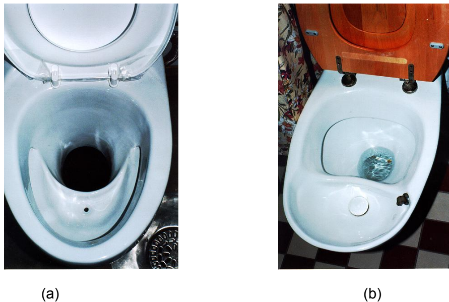
Figure 2.11: Swedish urine-diversion pedestals for (a) dry system and (b) flushing system. (Austin and Duncker 2002)
