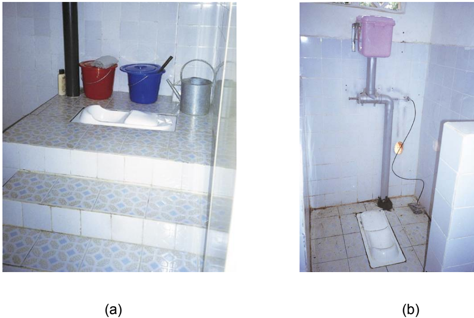
Figure 2.14. Urine-diversion ecosan toilets in Nanning area, China.
