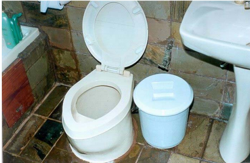
Figure 2.27: Retrofitted urine-diversion toilet in Richard Holden's house in Bellevue, Johannesburg (Photograph: CSIR)
