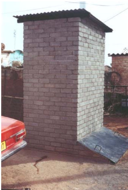
Figure 2.23: Toilets in Hanover, Northern Cape, are constructed with alternating drop-holes for the pedestal, but with a single vault. (Photographs: CSIR)
