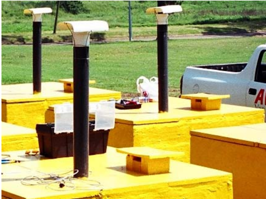
Figure 5.5: Ventilation of vault
