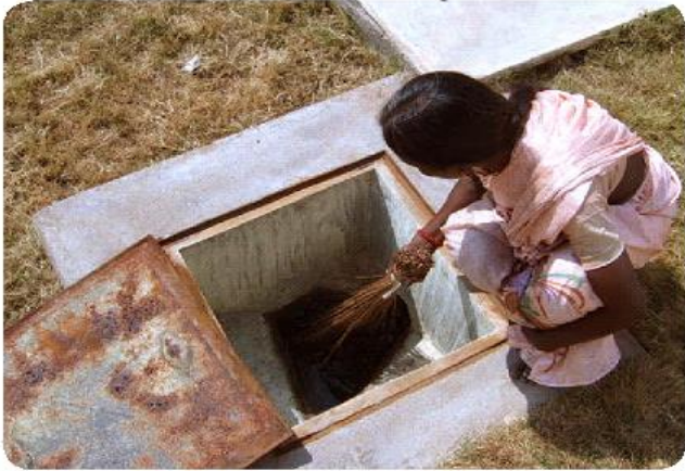
Cleaning of inspection chambers
