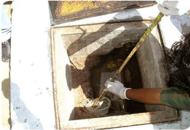
Removal of obstacle from the sewer pipeline
