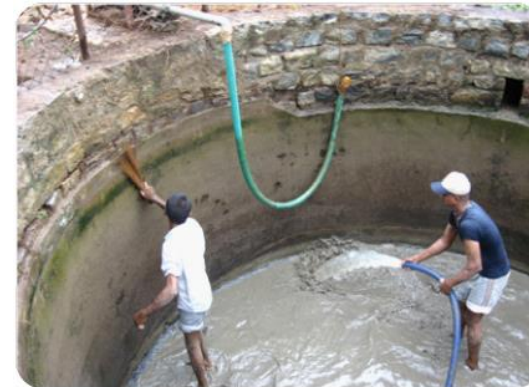
Cleaning the collection tank
