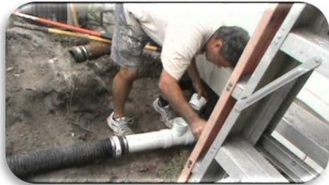
Replacement of pipes
