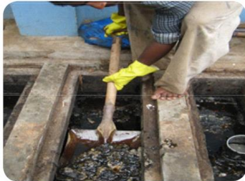
Removal of scum
