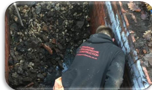
Cleaning and replacement of filter material
