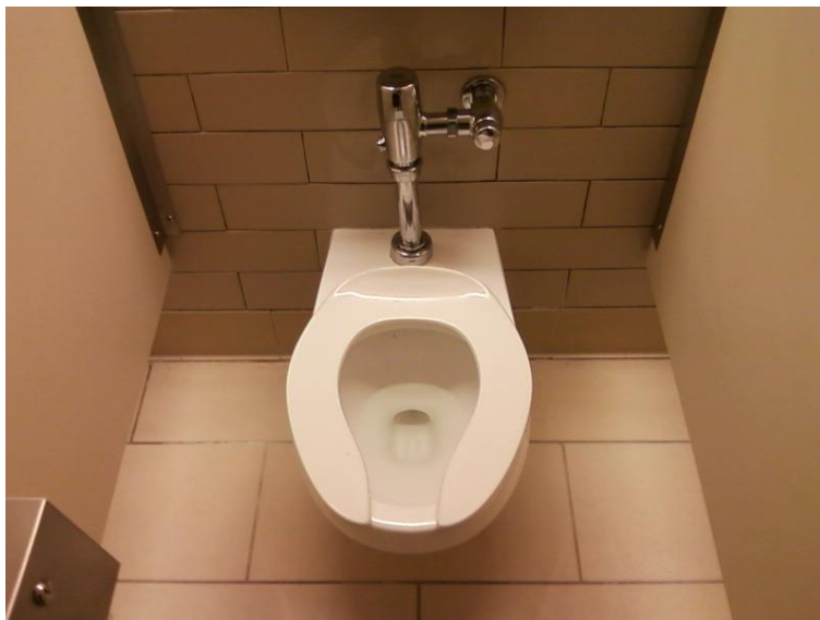
Figure 9: Typical public toilet using a demand flush at the Aquaduct Racetrack Casino (Bestway64 2012)
