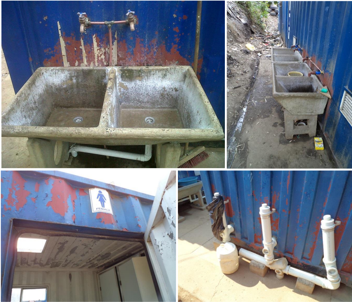
Figure 15: Photographic evidence of external paint requiring repair
