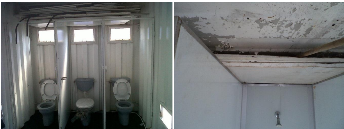
Figure 13: Photographic evidence of the storage of the cubicle doors
