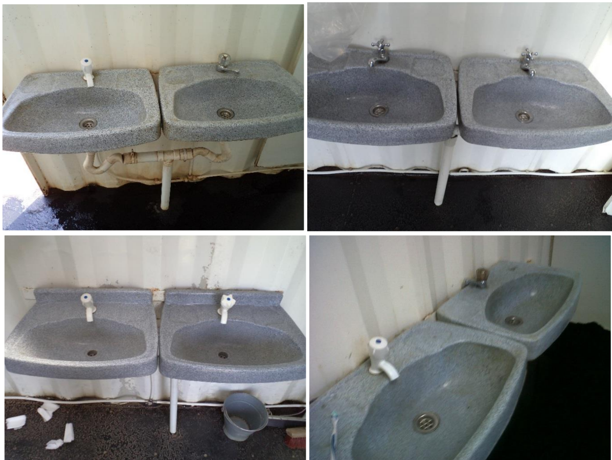
Figure 19: The wash hand basin taps turning
