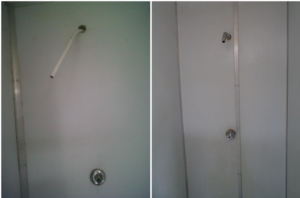
Figure 17: The typical configuration of a shower without a shower head
