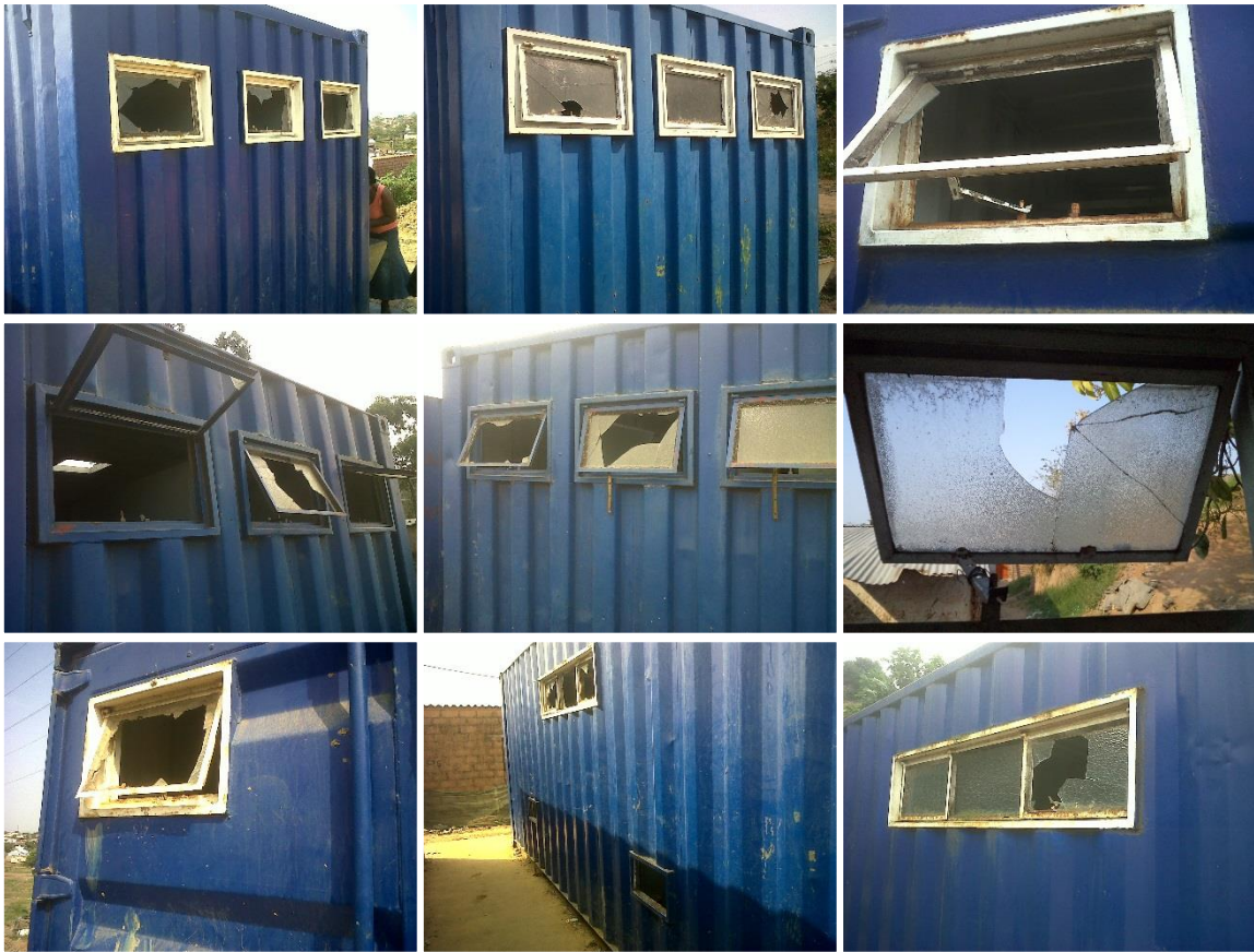
Figure 6: Evidence of the type of broken windows found at the CAB sites
