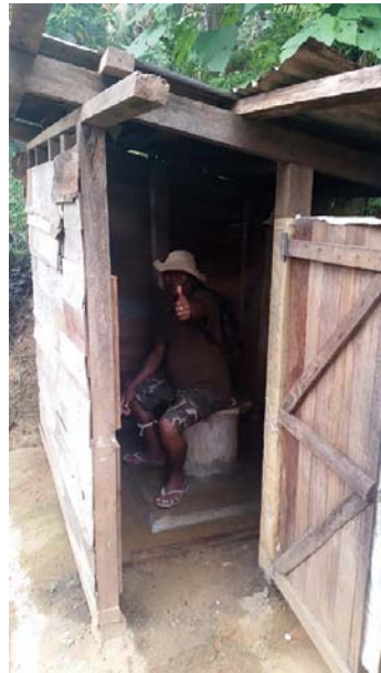
White River Settlement – New latrine
