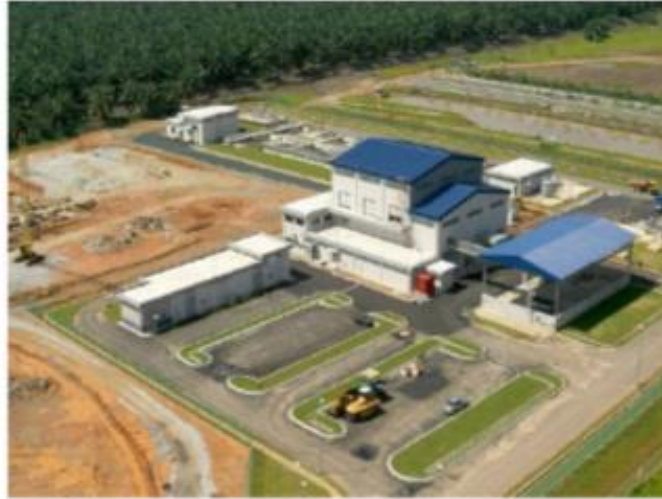
Centralised Sludge Treatment Facility
