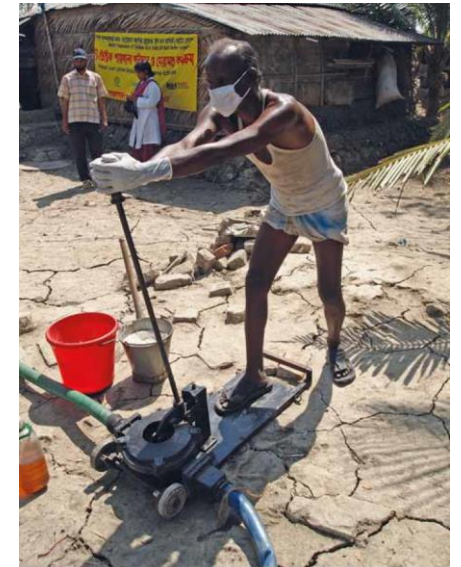
Figure 4.7 Manual diaphragm pump operation in Bangladesh (photo: Georges Mikhael).
