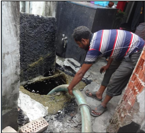
Emptying by vaccum pump (< 100 m sucking pipe) and truck
