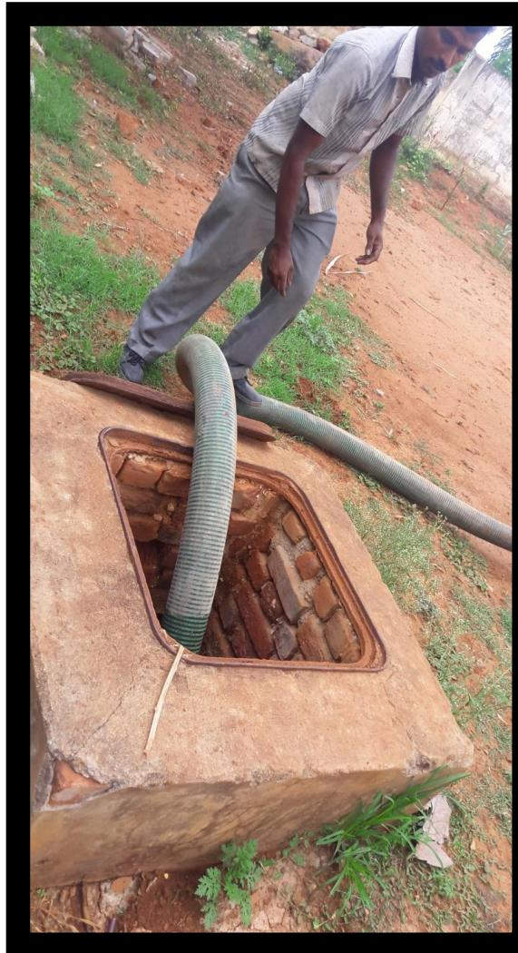
However a small amount of sludge should be left in the tank to ensure that a minimum level of the necessary microorganisms responsible for anaerobic digestion remain in the tank
