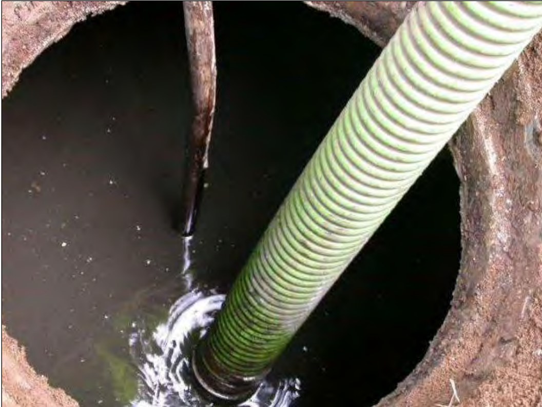
Figure 9: Cleaning of interceptor tank
