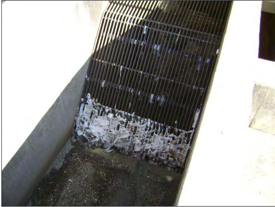
Figure 18: Manual screening with rake
