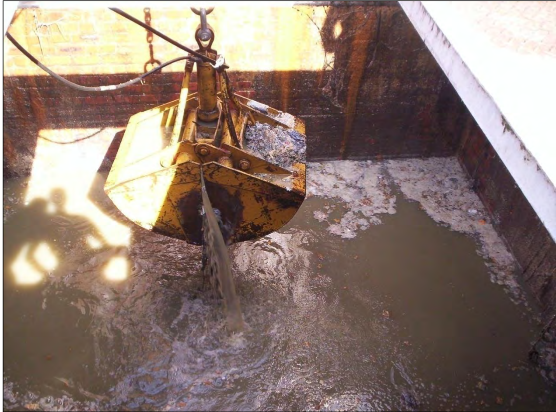
Figure 13: Grapple bucket removing silt in Gugulethu (courtesy of BKS (Pty) Ltd)
