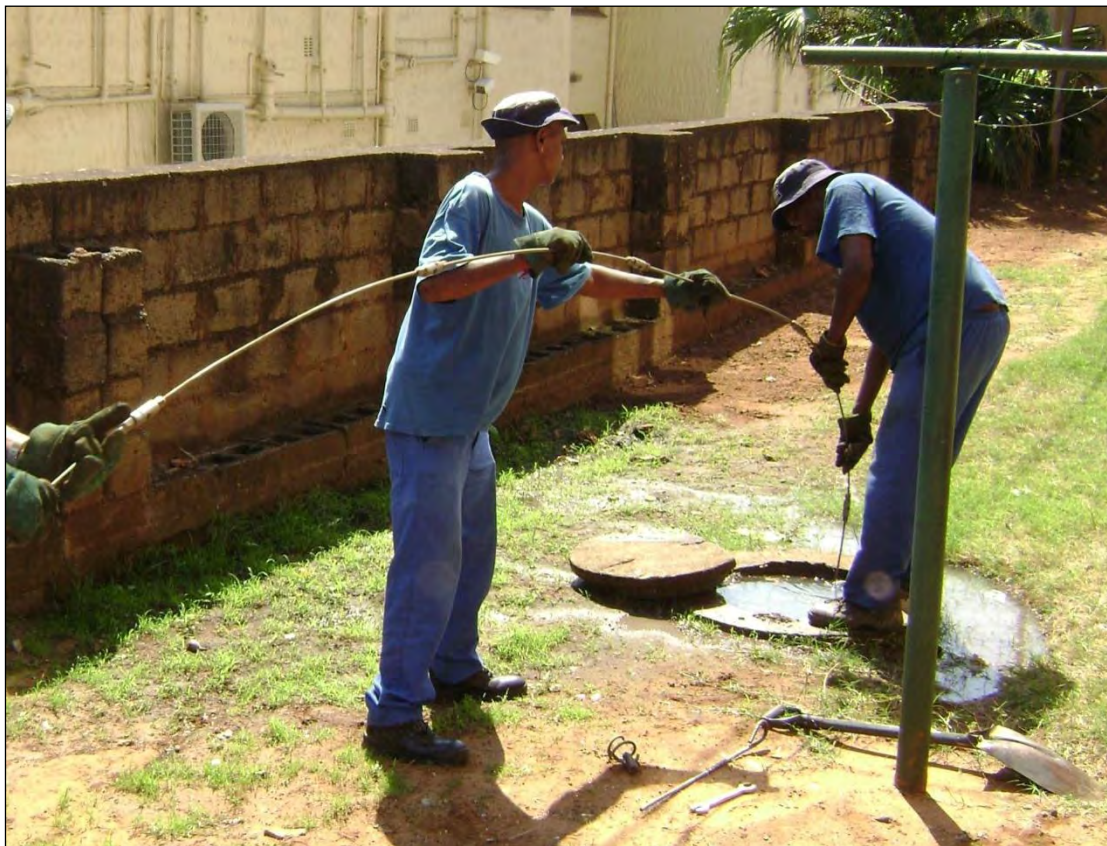
Figure 2: Rodding of a sewer pipe
