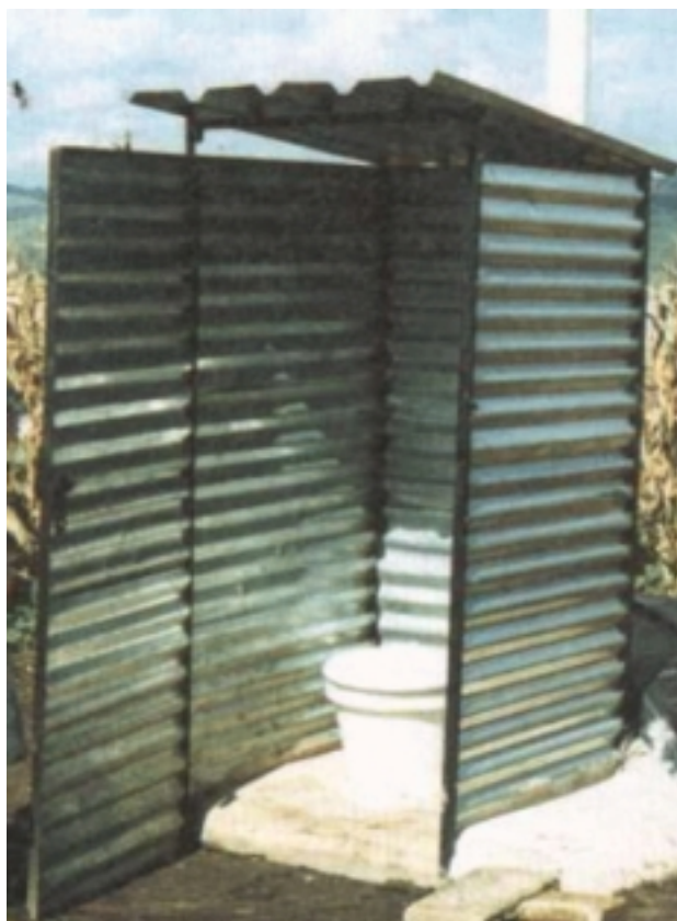
Figure 2: The VIP with a steel frame superstructure is a common solution to the problem of low cost and fast sanitation delivery. However, due to cost considerations these structures tend to be cramped. Also the fly control and odour control design features of a true VIP are not observed.
