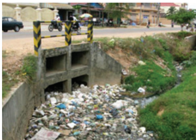
Solid waste management is essential if drainage is to function
