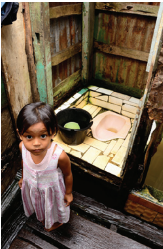
Despite the presence of a basic, though hygienic, communal toilets located a few meters away, users often value privacy and convenience over downstream consequences. This latrine in Palembang, Indonesia, looks quite nice; however, it discharges directly into the river.
