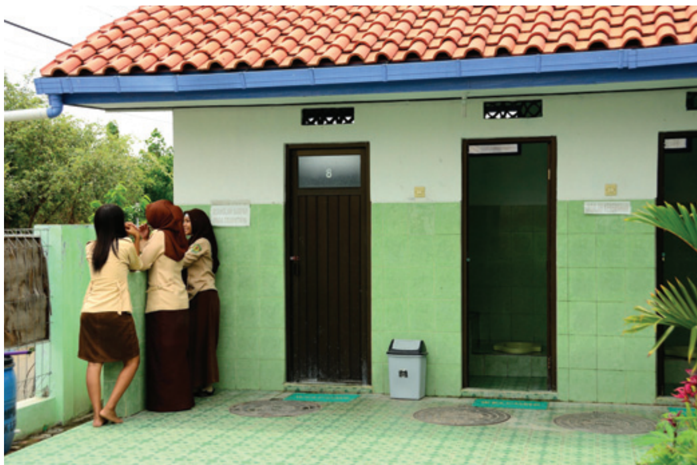
Well-maintained communal toilets and septic tank system developed by Care International in Makassar, South Sulawesi, Indonesia.
