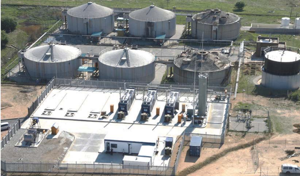
Figure 15: View of the NWWTW anaerobic digesters and CHP plant
