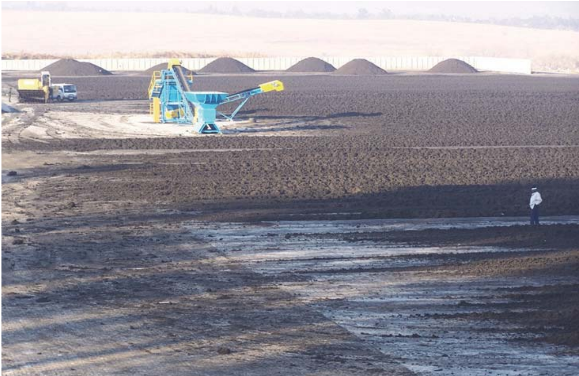
Figure 21: Open air solar drying at the NWWTW
