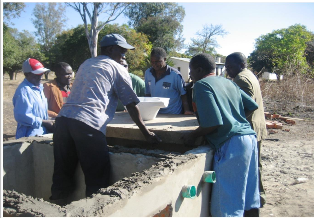
Placing of Slab
