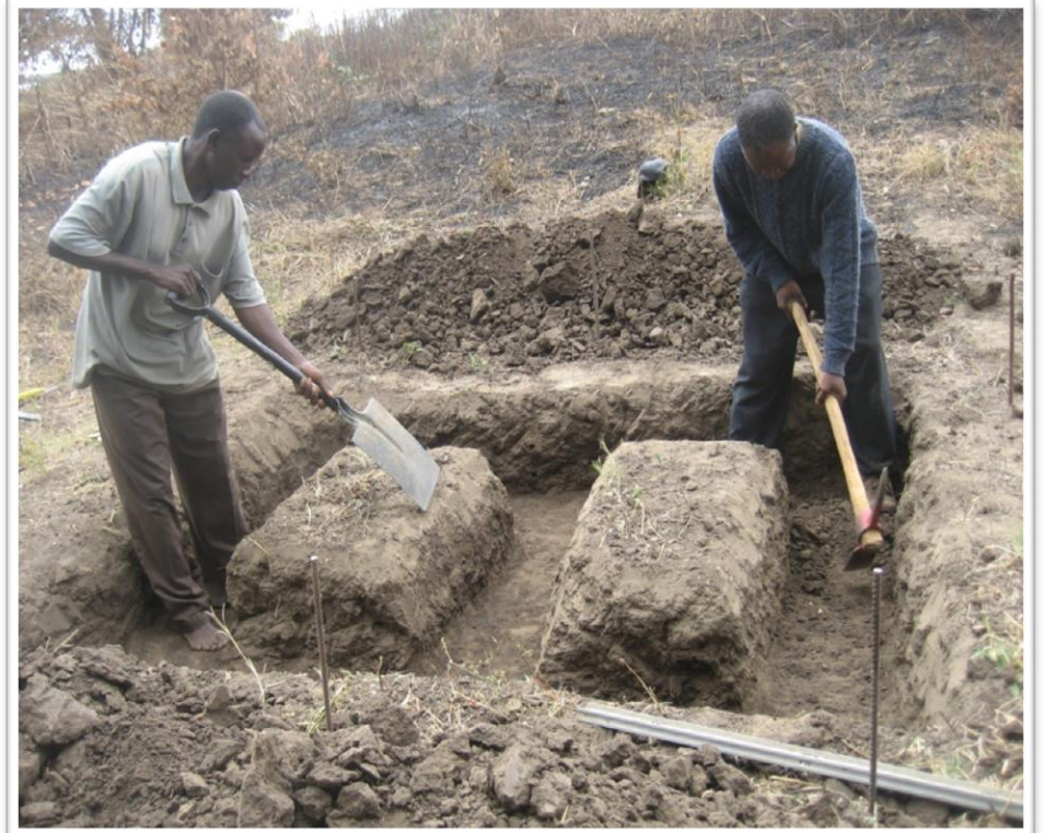
Lineout & Excavation
