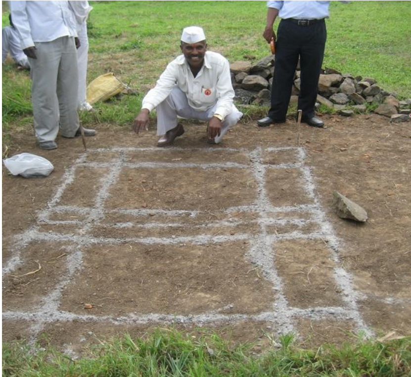
Lineout & Excavation
