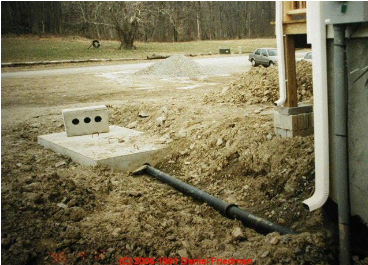
Piping and connecting to toilet pan
