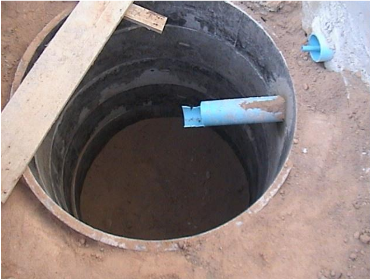
Pit Lined with concrete rings
