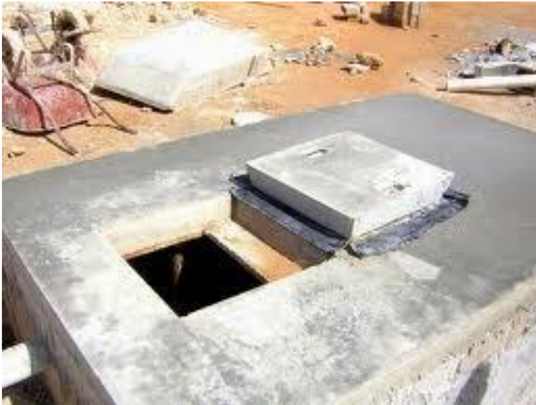
Cast roof with manhole and cover
