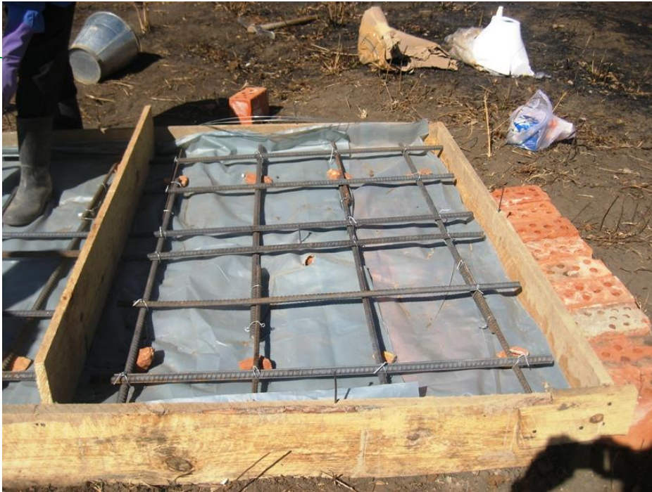
Slab Casting
