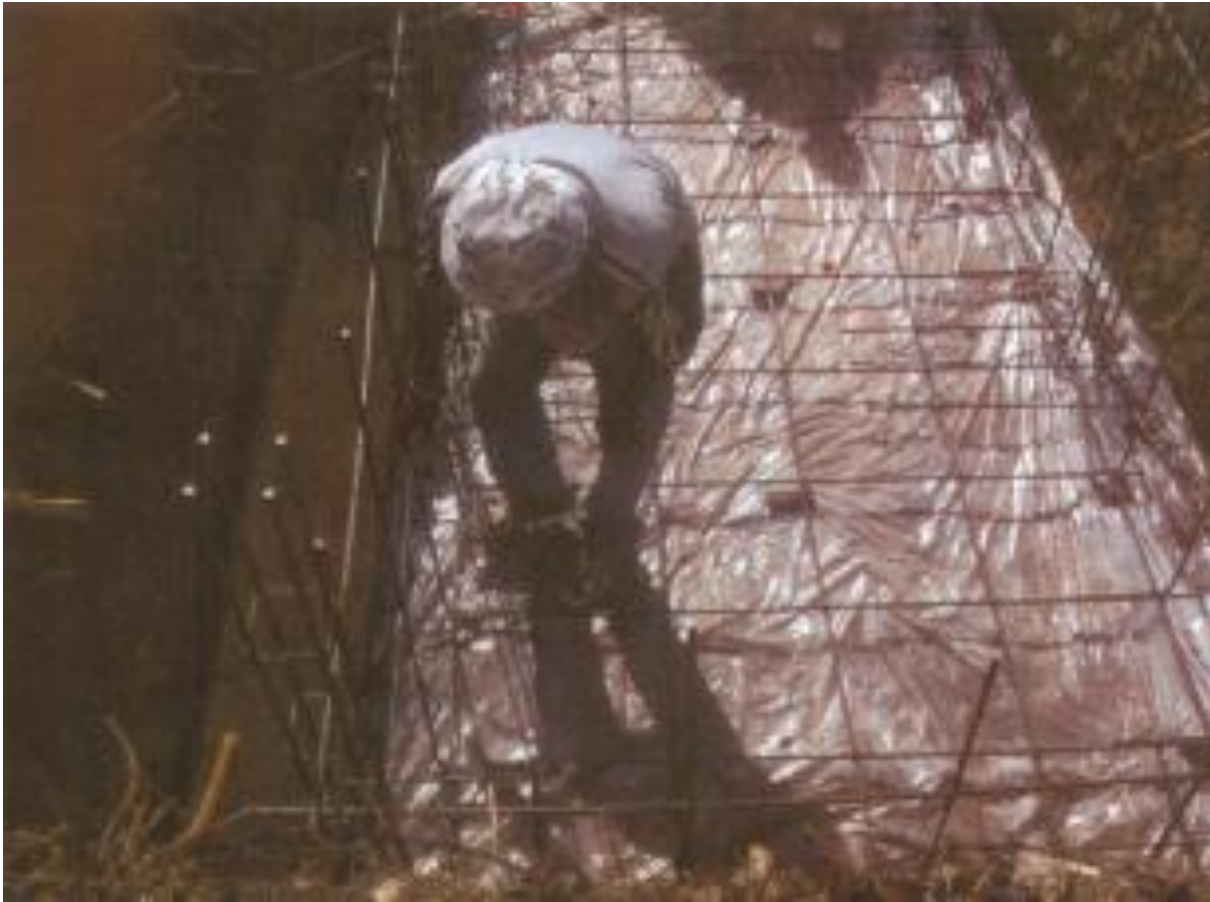
Base slab – Steel reinforcement
