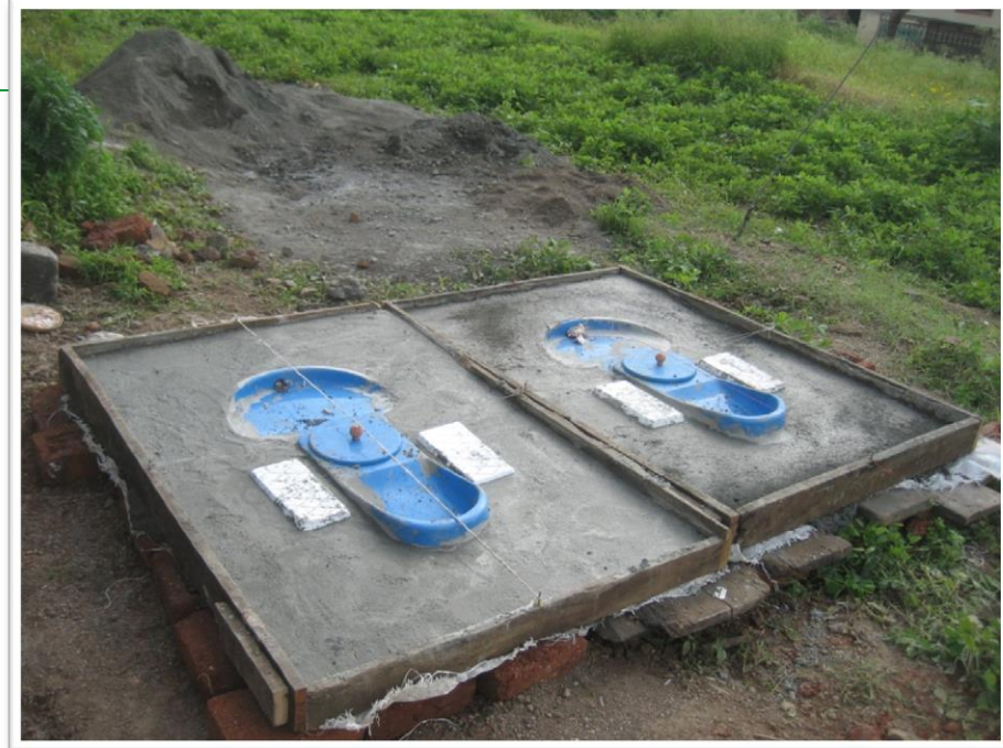
Slab Casting
