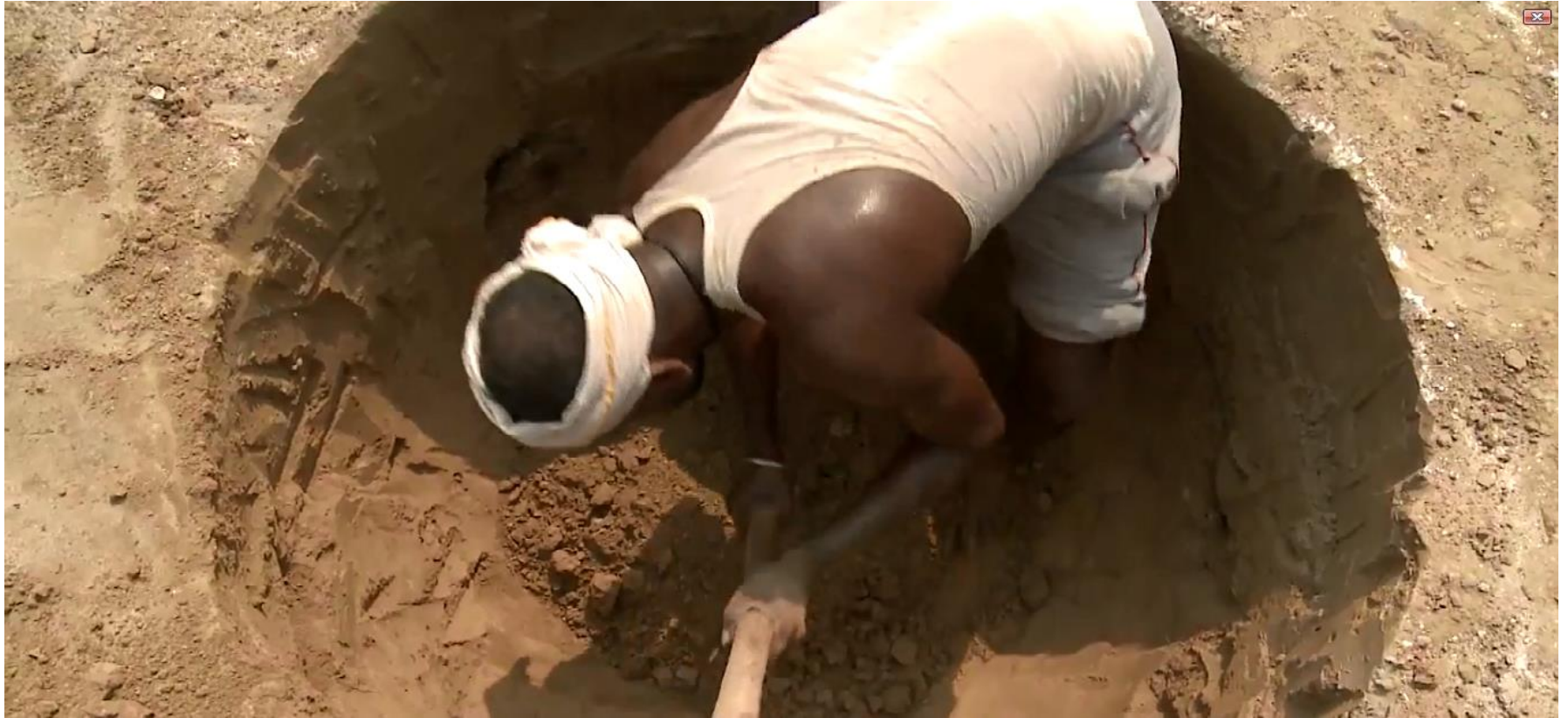
Excavation for the Pit
