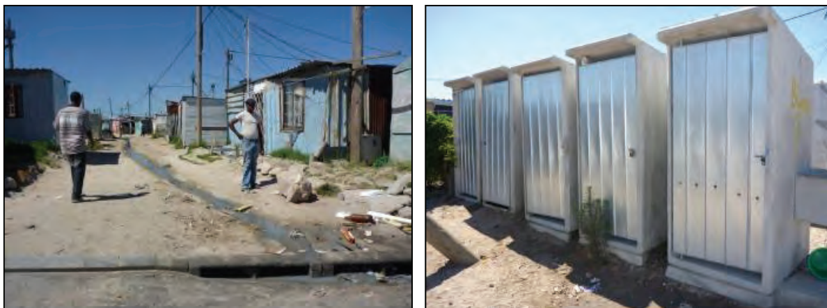
Figure 4-7: Open stormwater channel and drain (left) and communal toilets drained by vacuum sewer system (right) (Photos by Ashipala, July 2009).
