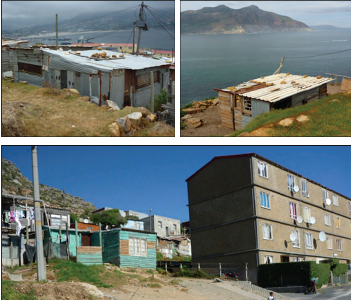
Figure 4-1: Photographs of Hangberg. From top clockwise: (a) dwellings located beneath the ‘sloot’ (ditch) with views overlooking the harbour, (b) a dwelling in neighbouring Dallas section and (c) informal dwellings built behind a row house (Photos by Taing, 2011).
