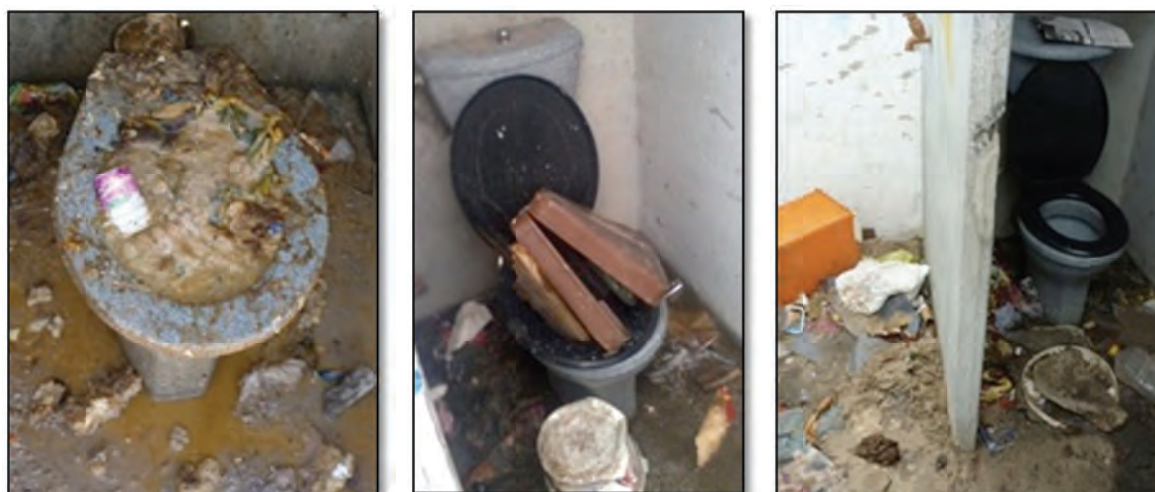
Figure 4-9: Evidence of greywater, food waste and solid waste disposal in Kosovo toilets connected to the vacuum sewer (Photos by Taing, 2010, 2011).
