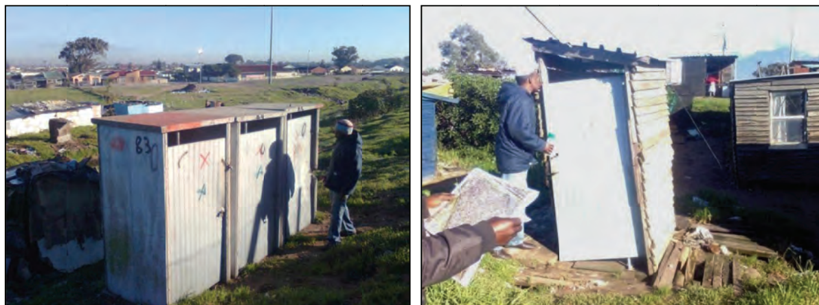
Figure 5-3: A row of communal container toilets (left) and a private pit latrine (right) (Photos by Ashipala and Pan, 2010).
