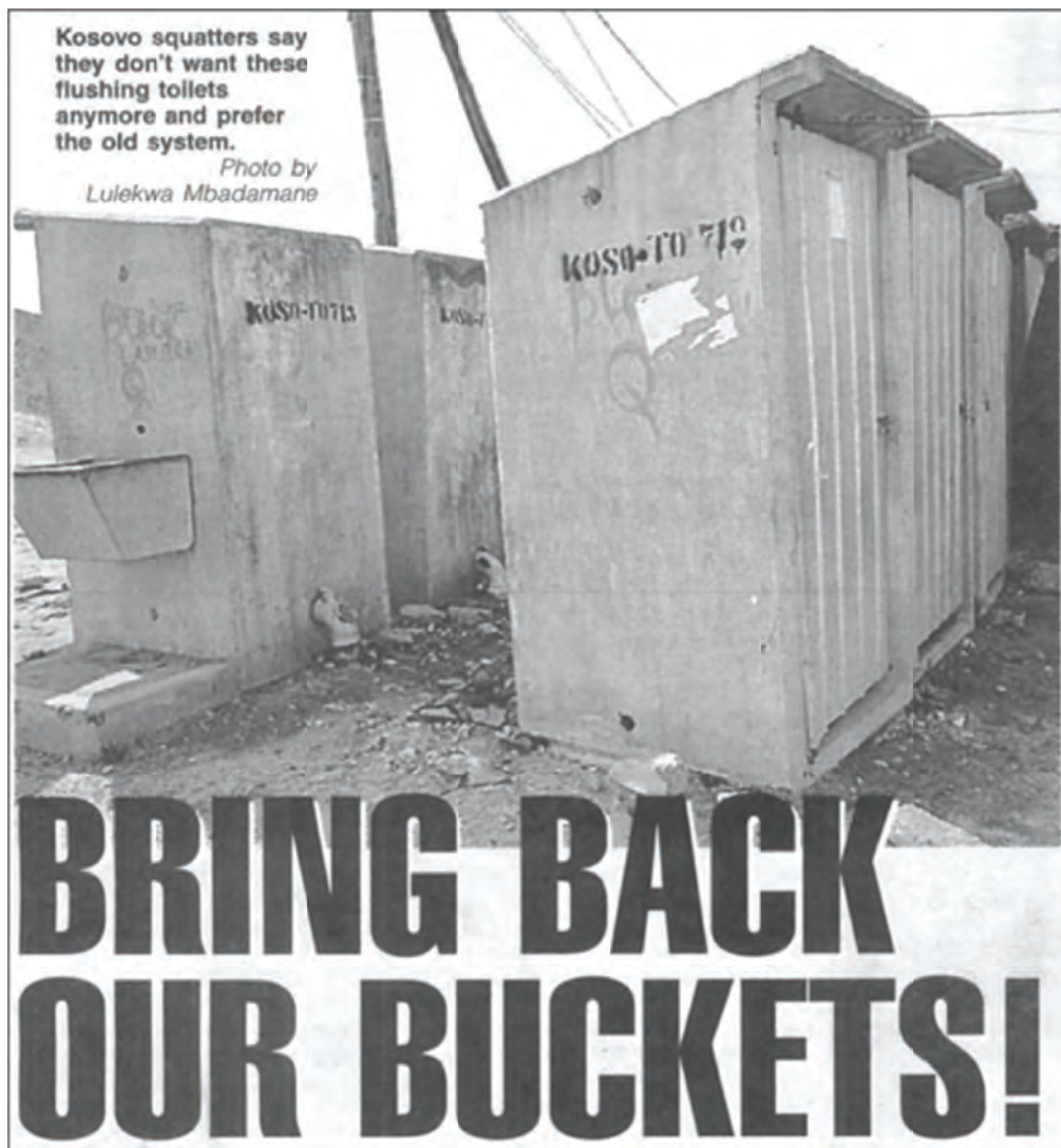
Figure 1-1: Daily Sun's (2011) coverage of Cape Town's vacuum sewerage system.
