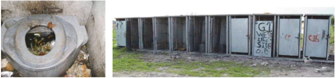
Figure 7: View of container toilets (source: Mels et al., 2008)
