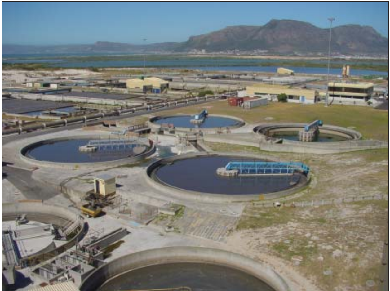
The Cape Flats Wastewater Treatment Works
