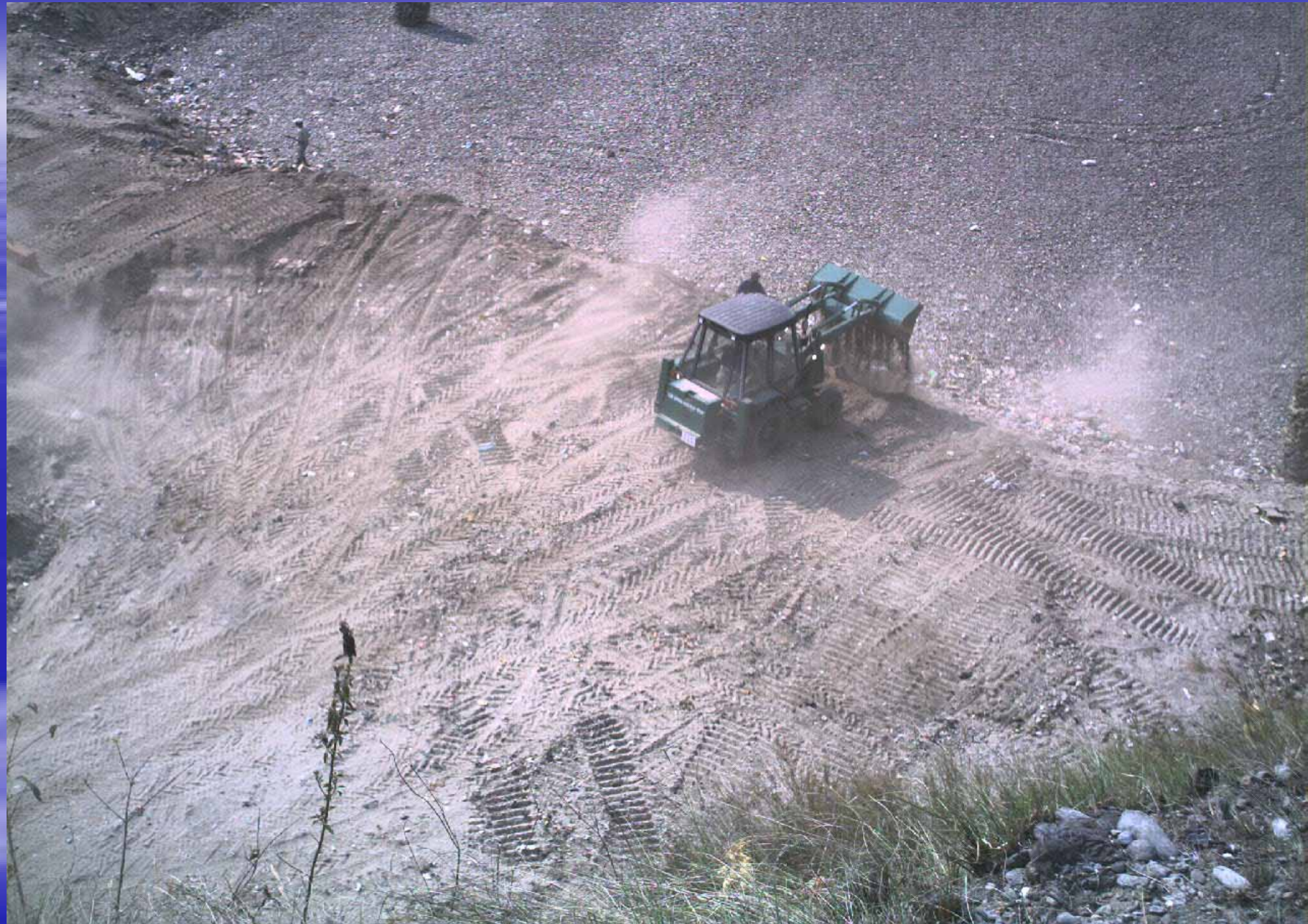
Soil spreading by loader
