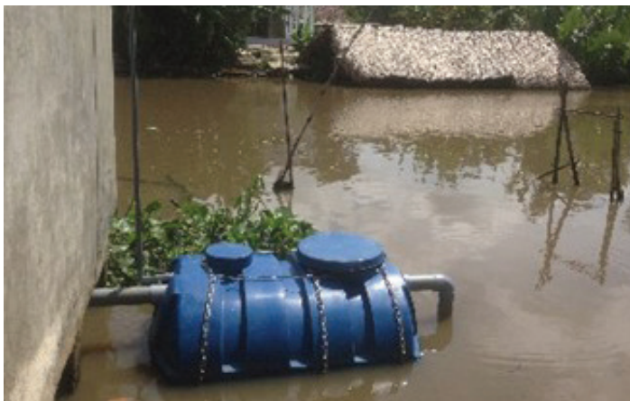
Figure 4. Plastic Septic Tanks for Flood-prone Areas
