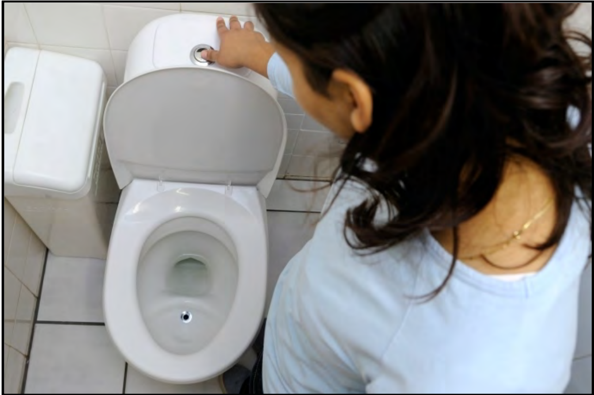
Figure 13 Overhead view of the No-Mix toilet showing a front compartment for urine separation and the back compartment for faecal waste as for standard toilets.
