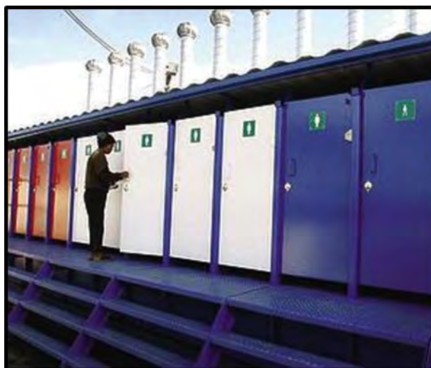
Figure 21 Dry urine diversion toilets (MobiSan prototype unit) at Pooke se Bos Informal Settlement in Cape Town.
