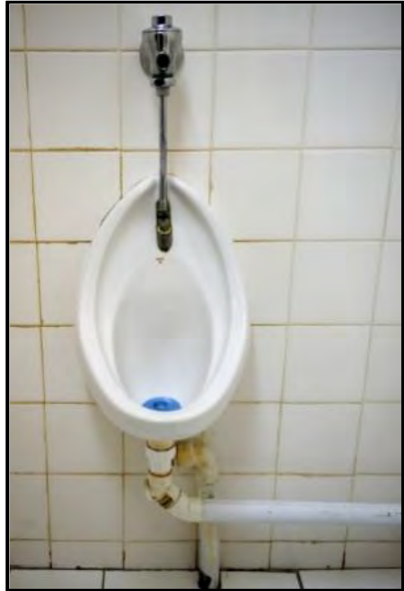
Figure 14 Urinals retrofitted with one-way waste valves which allow the urine to pass and prevent odours from escaping.
