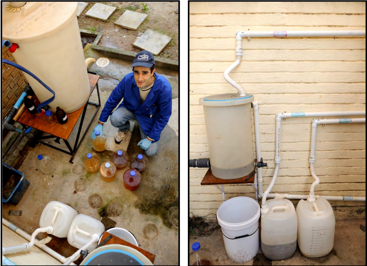
Figure 16 Waste stream collection and storage area in the courtyard outside the CSIR office block, with brown water collection tank and blue macerator pump line seen top left (left) and four urine collection tanks 40 l ladies' no-mix urine, 25 l men's urinals and 25 l men's no-mix urine, plus overflow to sewer (right)
