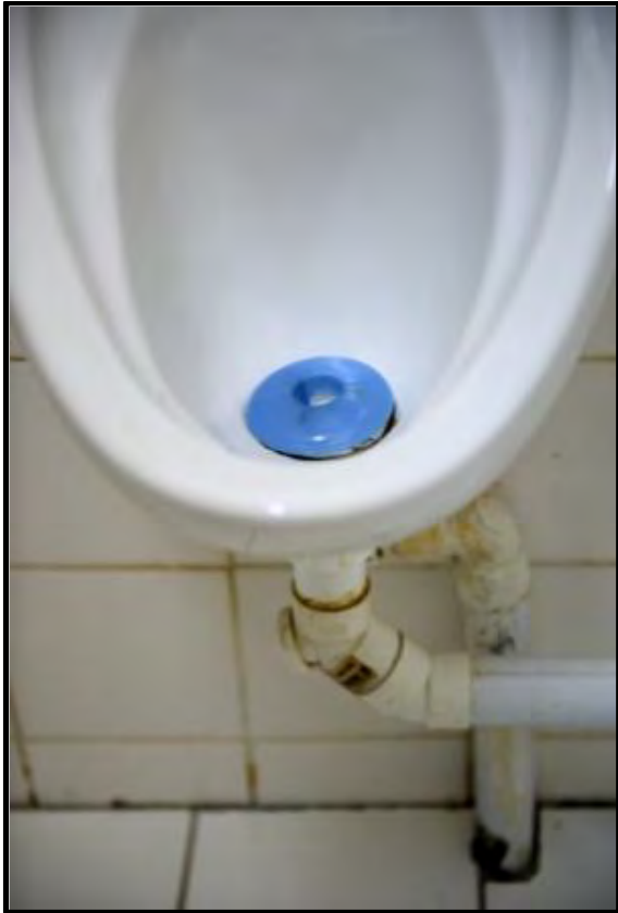
Figure 14 Urinals retrofitted with one-way waste valves which allow the urine to pass and prevent odours from escaping.
