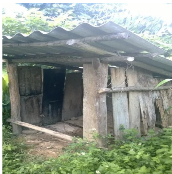
Pic 3. Dug hole latrine in Sa Long 1 hamlet
