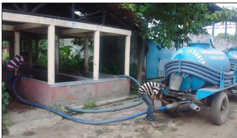
Figure 6: Disposal of Septage at FSTP facility
