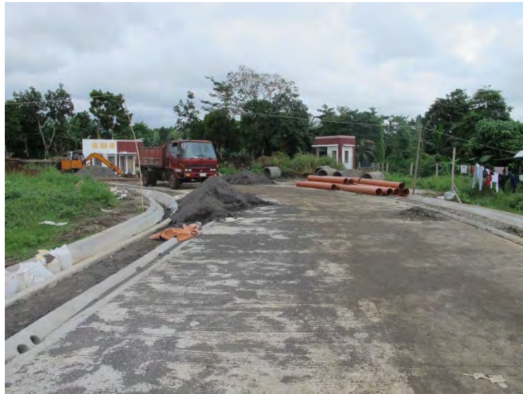
Figure 3: Construction of septage treatment facility
