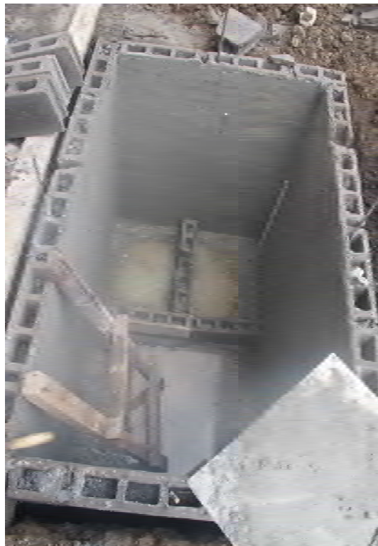
Figure 2: Septic tank under construction in Camella housing estate, Naga City
