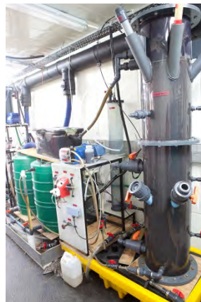
Urine processing reactors
