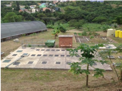
DEWATS plant and growing tunnel
