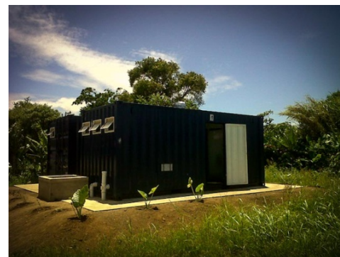
The CAB and the concrete enclosure used to house the water monitoring equipment, the water meters and data loggers.
