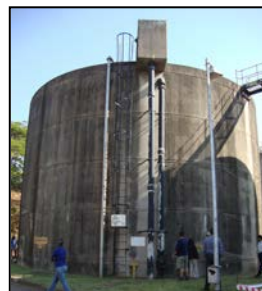
Full scale co-digester located at the Amanzimtoti Waste Water Treatment Works
