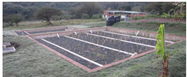
Fig.2: Vertical flow constructed wetland
