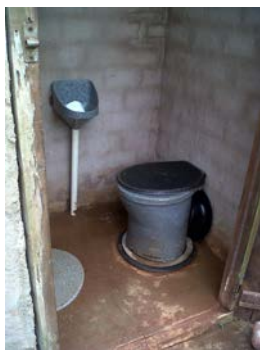
Inside view of UDT
