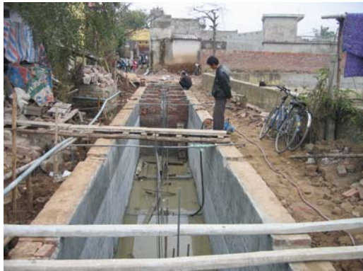
Figure 3. BASTAF under construction for a group of 80 households in Lai Xa commune, 20 km from Hanoi centre (photo by Nguyen V. A., 2006)
