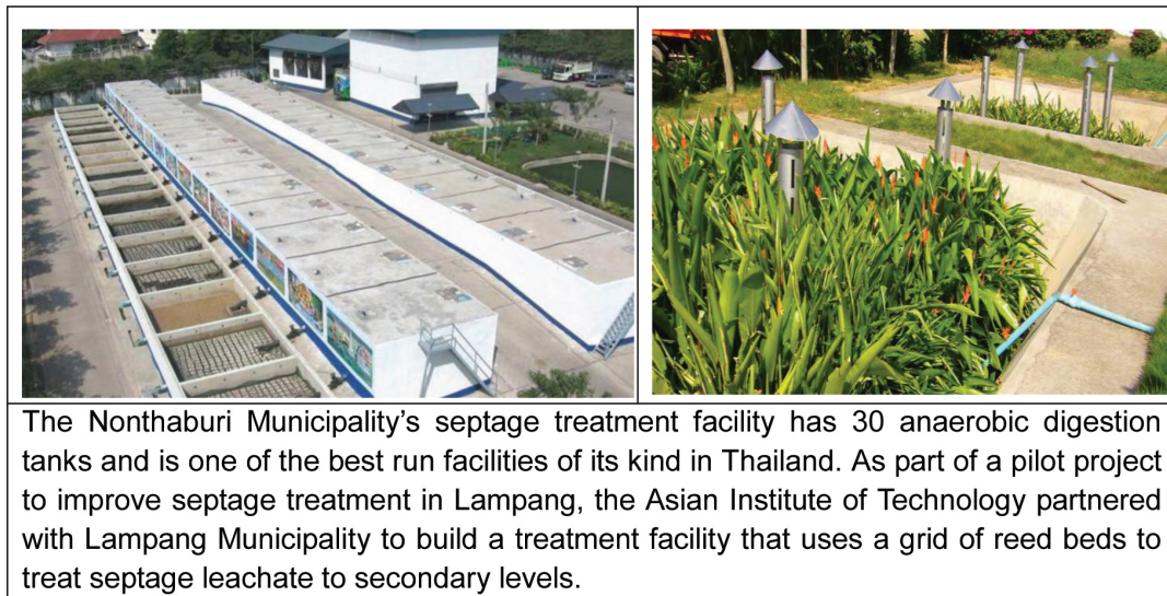
Figure 9.21 A photo view of septage treatment process at Nonthaburi in Thailand
