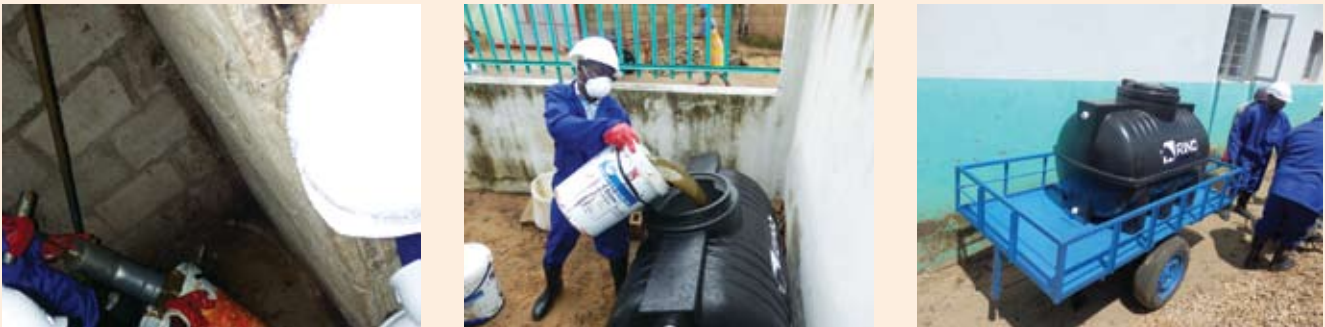
FIGURE 14: TRAINING SESSION ON EMPTYING AND TRANSPORT OF FECAL SLUDGE FROM PIT LATRINES
