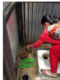
Chlorine (bleaching powder) being charged
