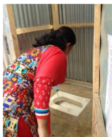
Bacterial mix being charged at a Enbiolet unit (flows into the first chamber)
