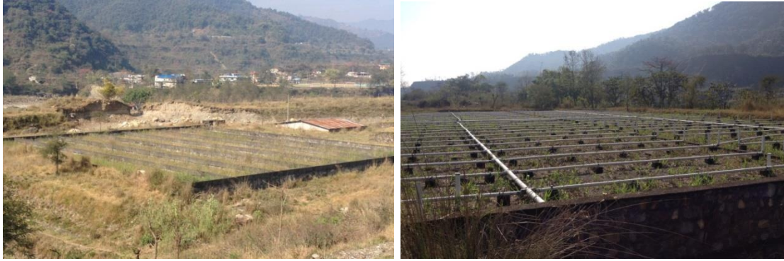
Figure 4: FSTP showing Sludge Drying Beds and Constructed Wetlands, Pokhara
