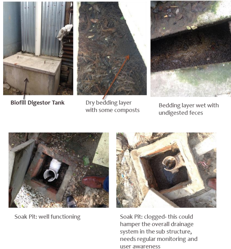
Figure 8: Biofill system under operation in Bangladesh
