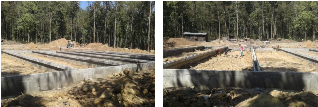
Figure 5: Sludge Drying Beds (under construction), Mukundapur, Nawalparasi
