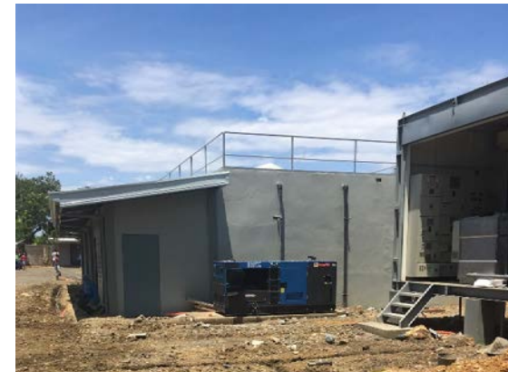
Top: Mechanical dewatering unit
