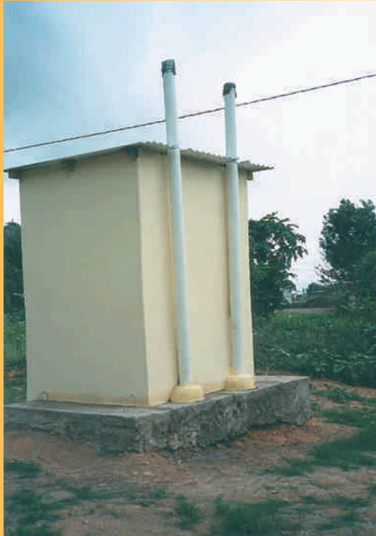
A Ventilated Improved Double Pit latrine - which is a dry sanitation system not requiring water for operation - is one of the options for construction.
