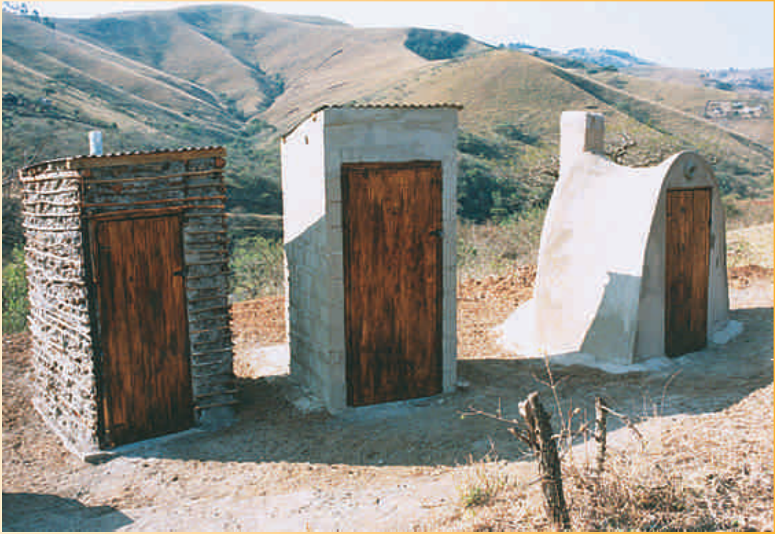
Communities are encouraged to use local resources and available building materials for the construction of structures for sanitation facilities.
