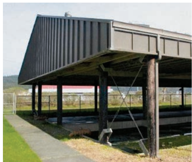
FIGURE 3. TYPICAL COVERED DRYING BED.
