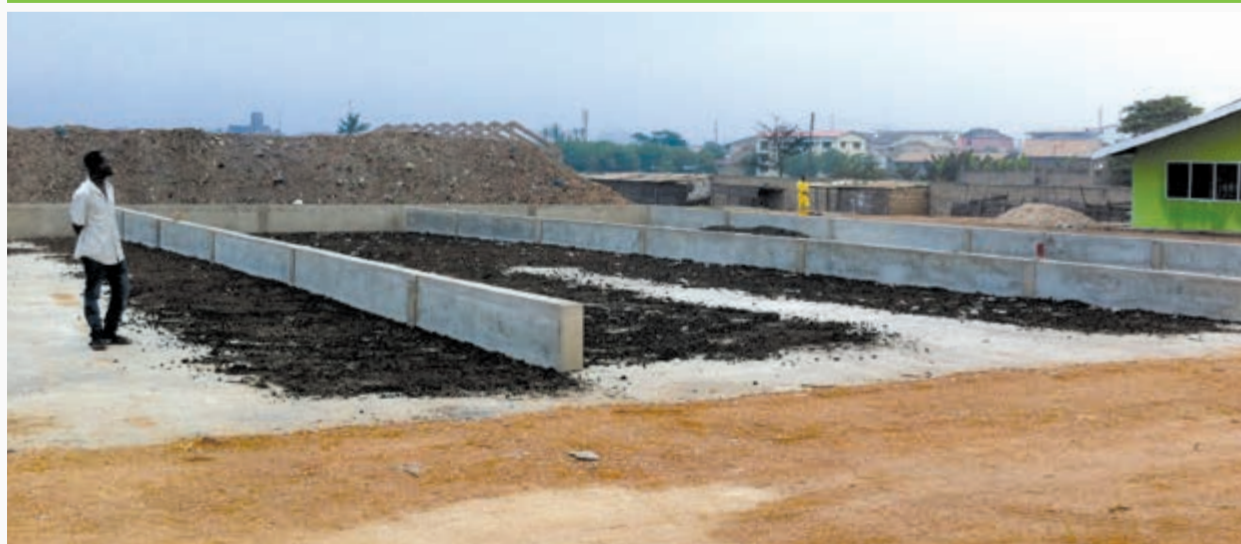
FIGURE 10. THE PAVED DRYING BEDS OF SLAMSON GHANA LTD., FS TREATMENT PLANT.
