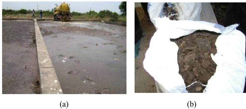
Plate S1. a) aseptic truck (capacity = 15 m 3 ) being emptied on the sand filter, and b) one bag of packaged DFS
