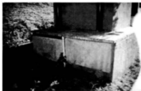
Figure 24: Photographs of UD toilets
