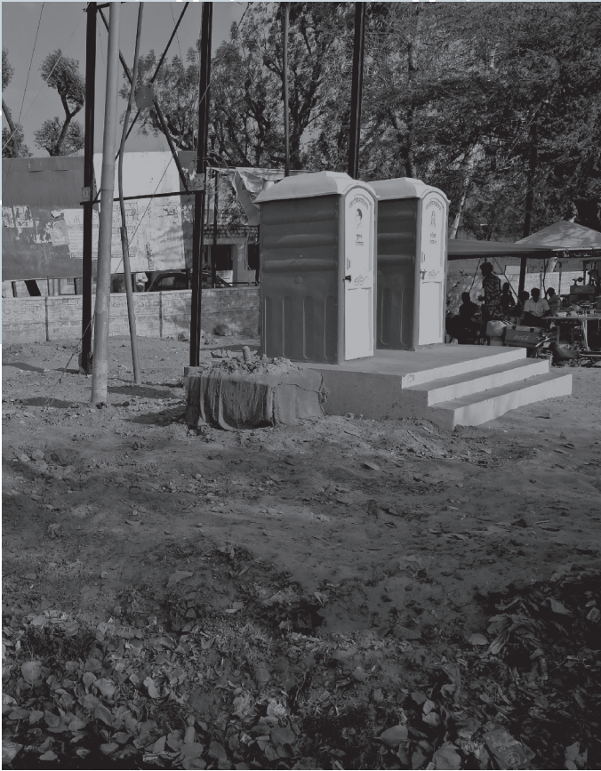
Figure 19: Public Toilet with Supernatant from OSS flowing into Open Drain
