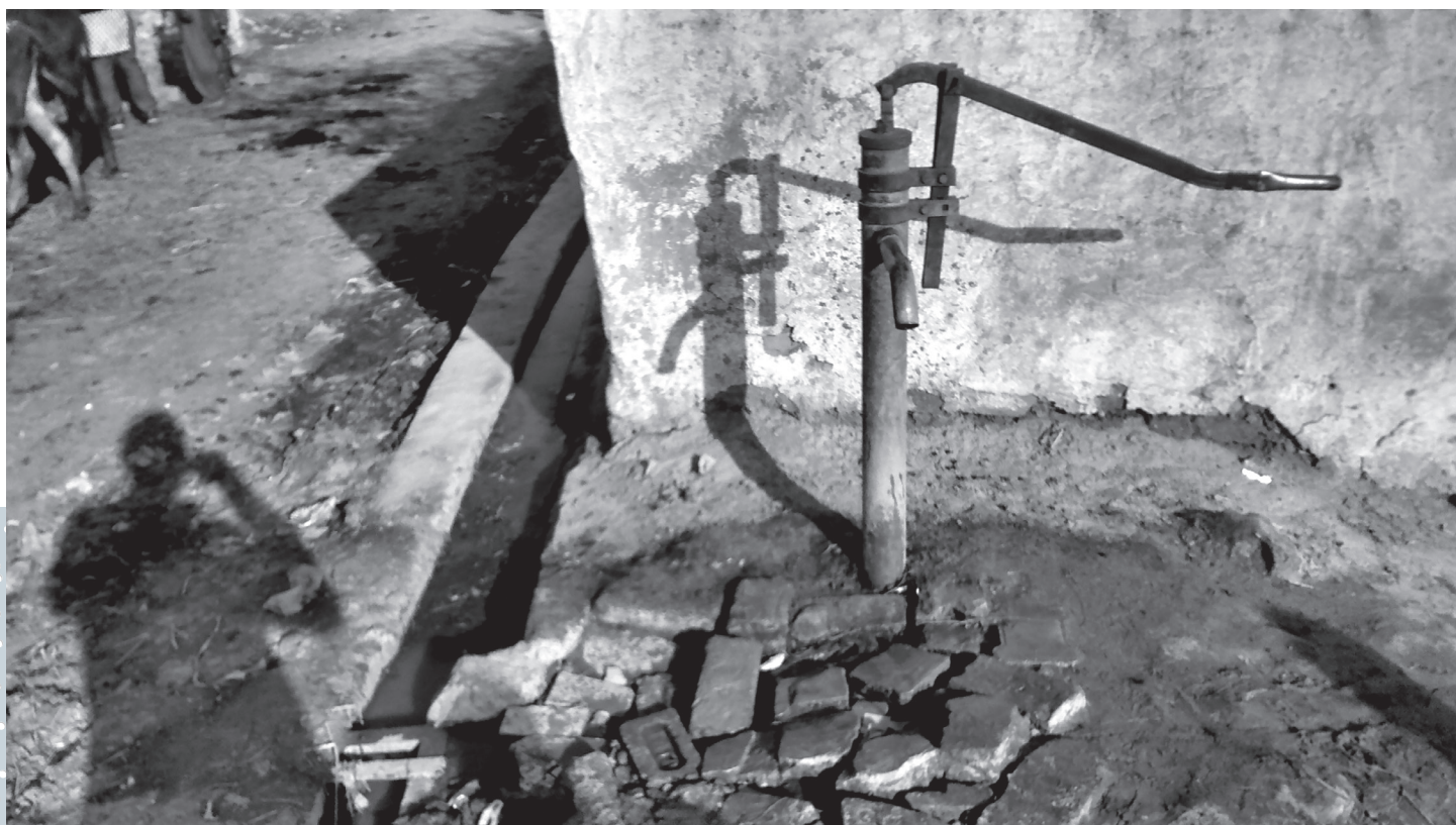
Figure 34: A Hand Pump Adjacent to a Drain at Risk of Contamination
