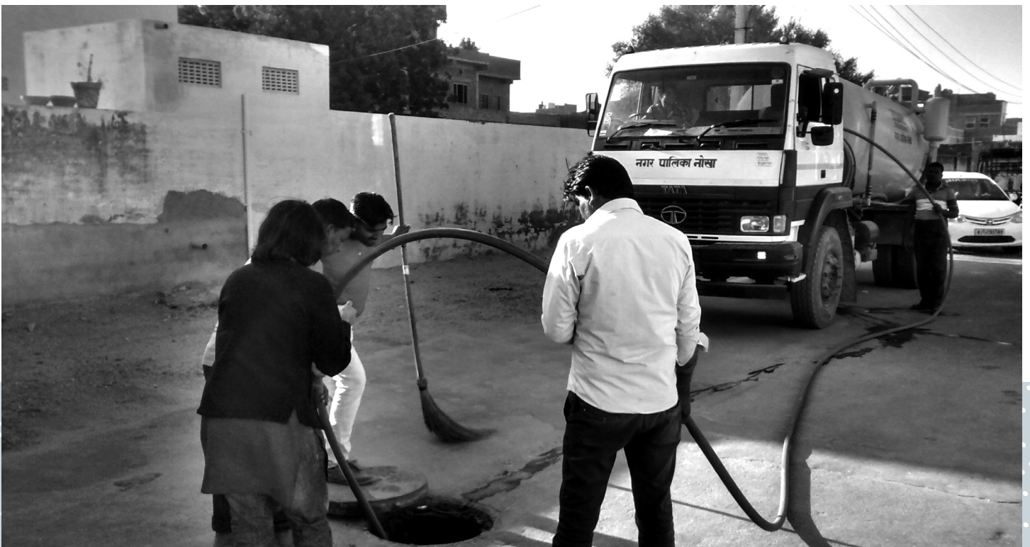
Figure 32: Desludging a Drain in Nokha to Remove Blockages Obstructing Wastewater Flow
