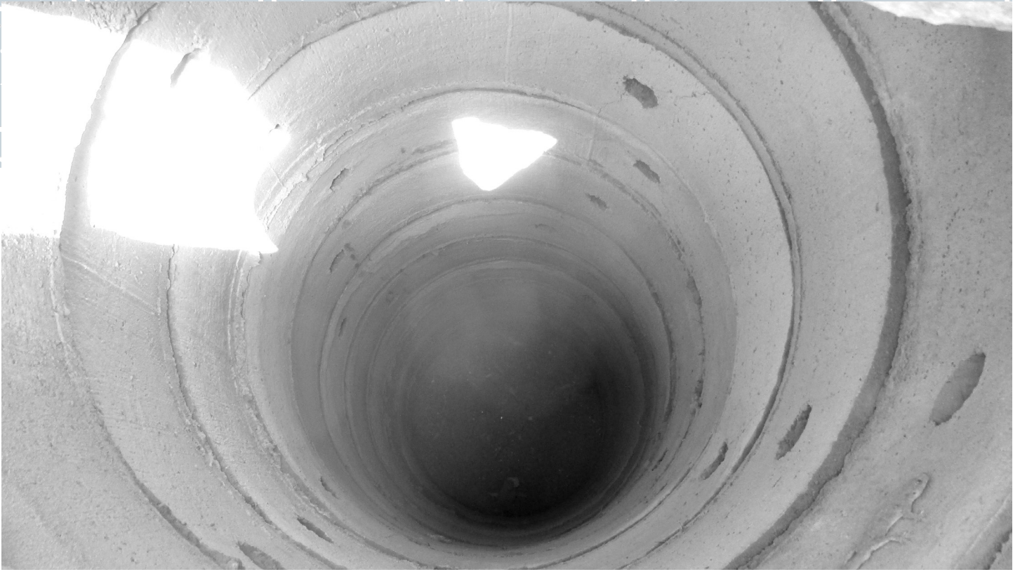
Figure 23: Unlined Pit (25 feet deep)
