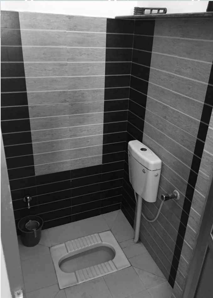
Figure 17: A Toilet with Cistern, Following the SBM Norms.
