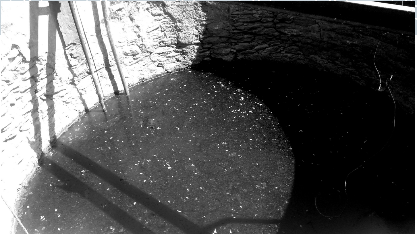
Figure 35: Water Percolating in a Well from a Nearby Polluted Lake Contaminating the Well
