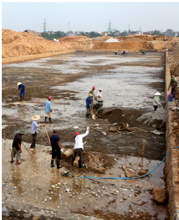
Constructing a centralized wastewater treatment facility in Thanh Hoa, Viet Nam
