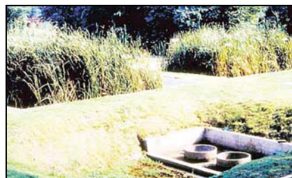
Photo 1: Cattail-planted constructed wetlands
