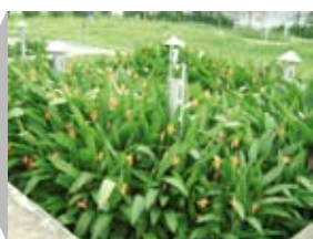
5) 2 nd Constructed wetland
