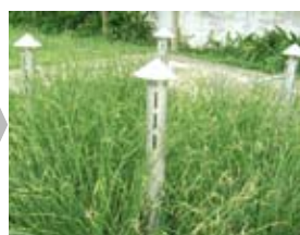
3) 1 st Constructed wetland
