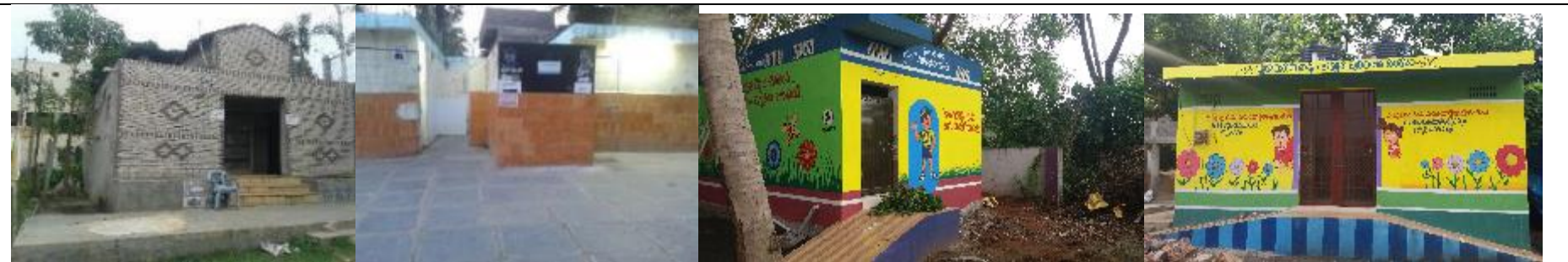
Photo 2-3 Public toilets in Kovvur
