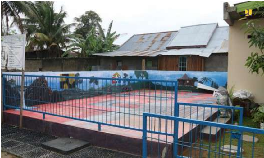
Community-based wastewater system uses a treatment unit that also require periodic sludge removal services. If agreed, they can also be the target of the scheduled desludging service.
