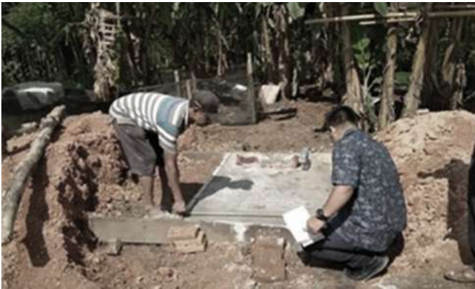
The municipality needs to regularly inspect every septic tank in its area, particularly to find out the condition, the utilization and the last desludging conducted. It is also necessary for the municipality to check on under-construction septic tanks.
