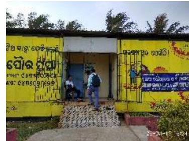
Figure 6: Public Toilet and its containment system in Puri
